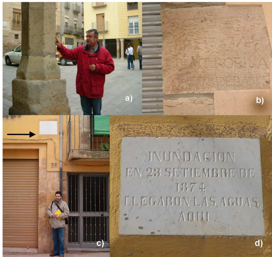
Figure 3.4. Three of the five limnimarks found: (a) carving on a column at Sant Antoni Square marking the 1644 flood's maximum water height (observation 2 in Fig. 3.5), (b) sandstone plaque at Sant Agustí Street corresponding to the 1783 flood (observation 3 in Fig. 3.5), (c) marble plaque (marked by an arrow) at Sant Agustí Street corresponding to the 1874 flood (observation 5a in Fig. 3.5) and (d) detail of that plaque
