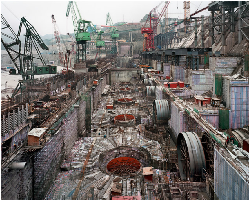
Dam #6 Three Gorges Dam Project, Yangtze River, China, 2005
