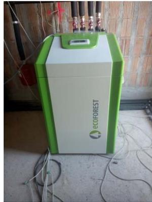
Figure 18. Geothermal heat pump
