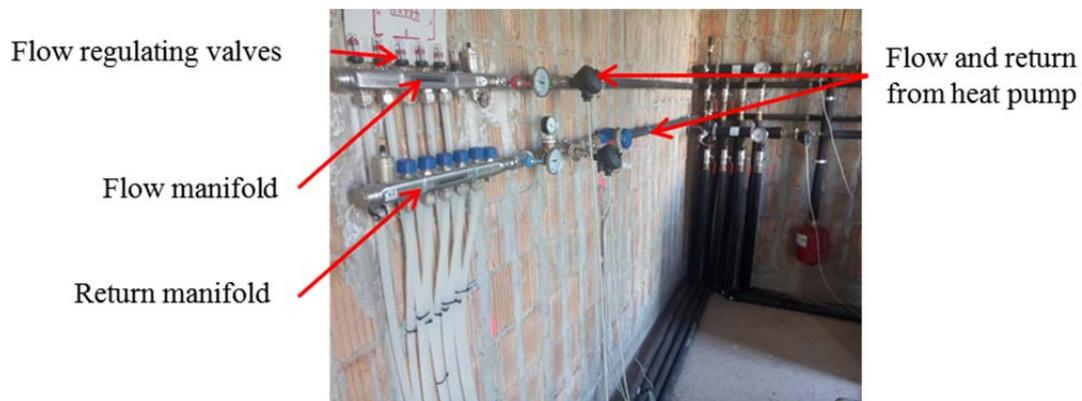
Figure 15. Radiant wall hydraulic connections
