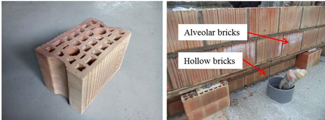
Figure 11. Sample of alveolar brick (left) and structure of the wall (right)
