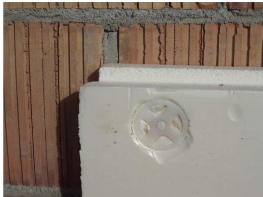
Figure 12. Hold of the insulation panels
