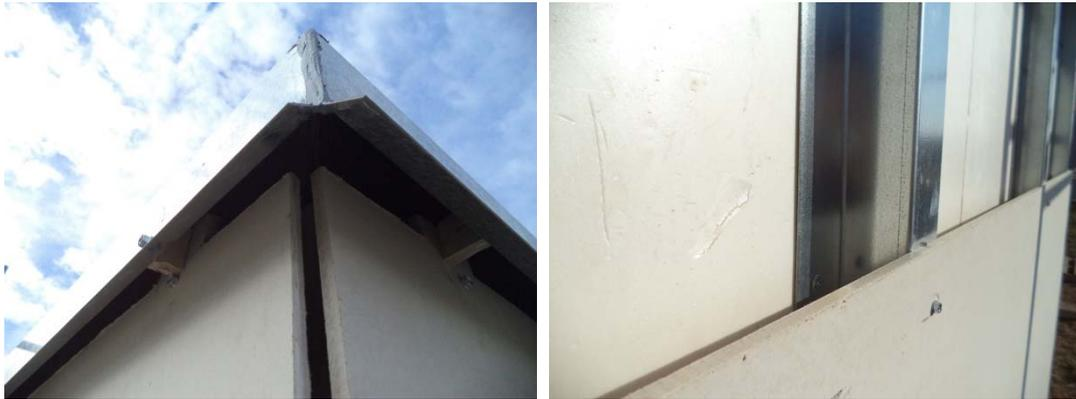
Figure 16. Details of the ventilated facade, structure (left) and top corner (right)
