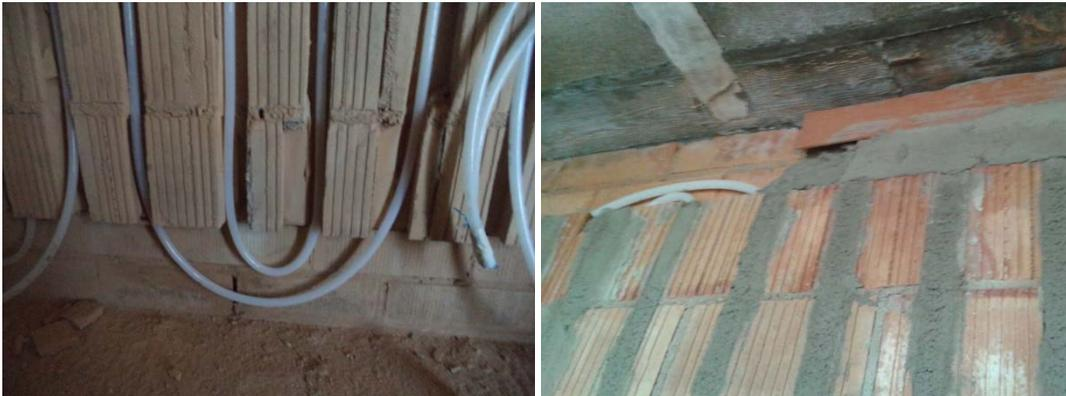
Figure 13. Pipes on groove before and during concreting (left and right respectively)
