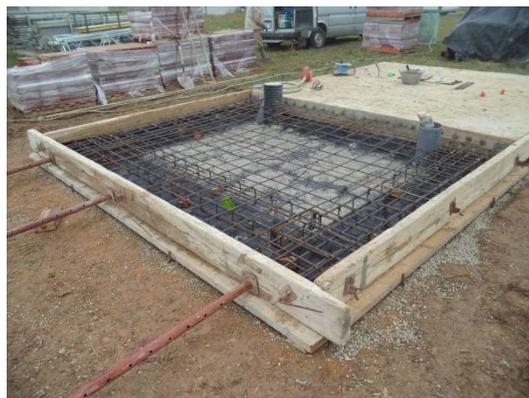
Figure 9. Concrete base during the construction process
