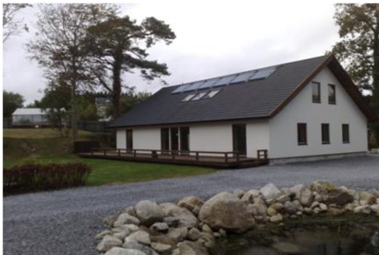
Fig. IV-2. Passive house in Galway (Ireland).
