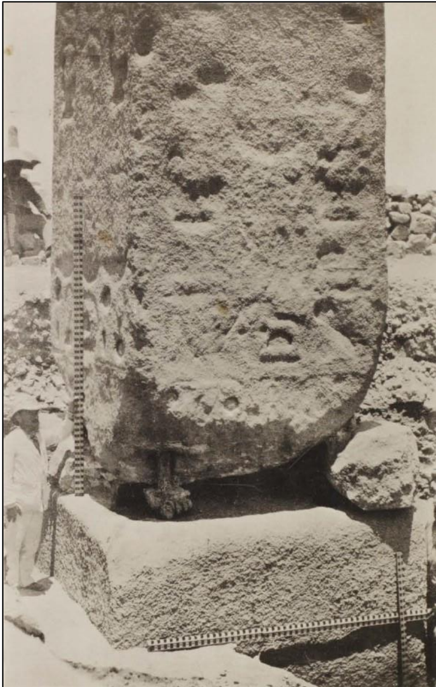
el-Ramleh. Le Hotel Métropole. Excavations revealing steps, pedestal, and position of crabs (Site 93. Gorringe 1885: Plate IV)
