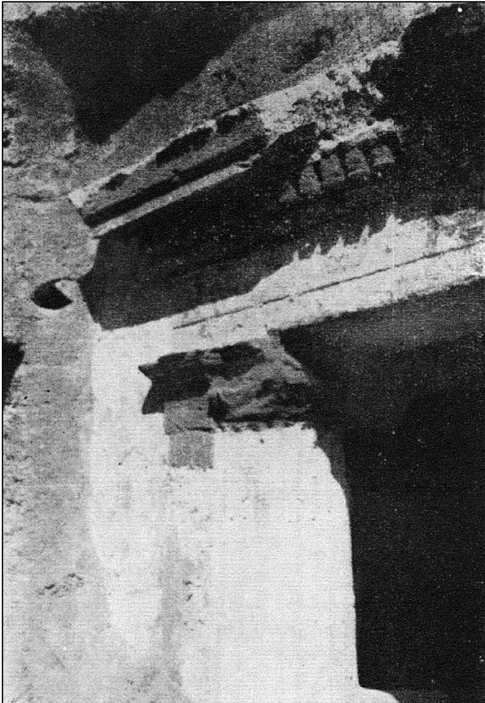
Minet el-Bassal necropolis. Sezione (A). Hypogeum (III) Façade of the κλίνη-alcove (Site 46. Adriani 1956a: 22, Fig. 23)
