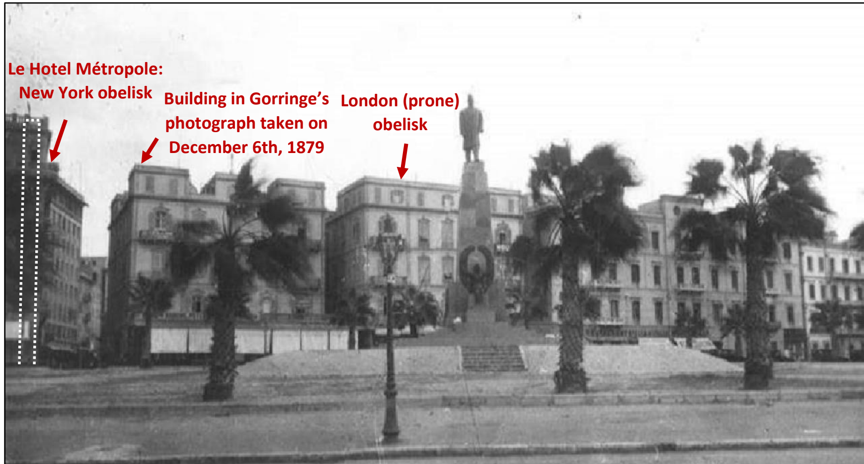
el-Ramleh. Saad Zaghloul Square. Le Hotel Métropole and buildings west of it Localisation of the Heliopolis obelisks (Site 93. pinterest.co.uk . Labels added by author)
