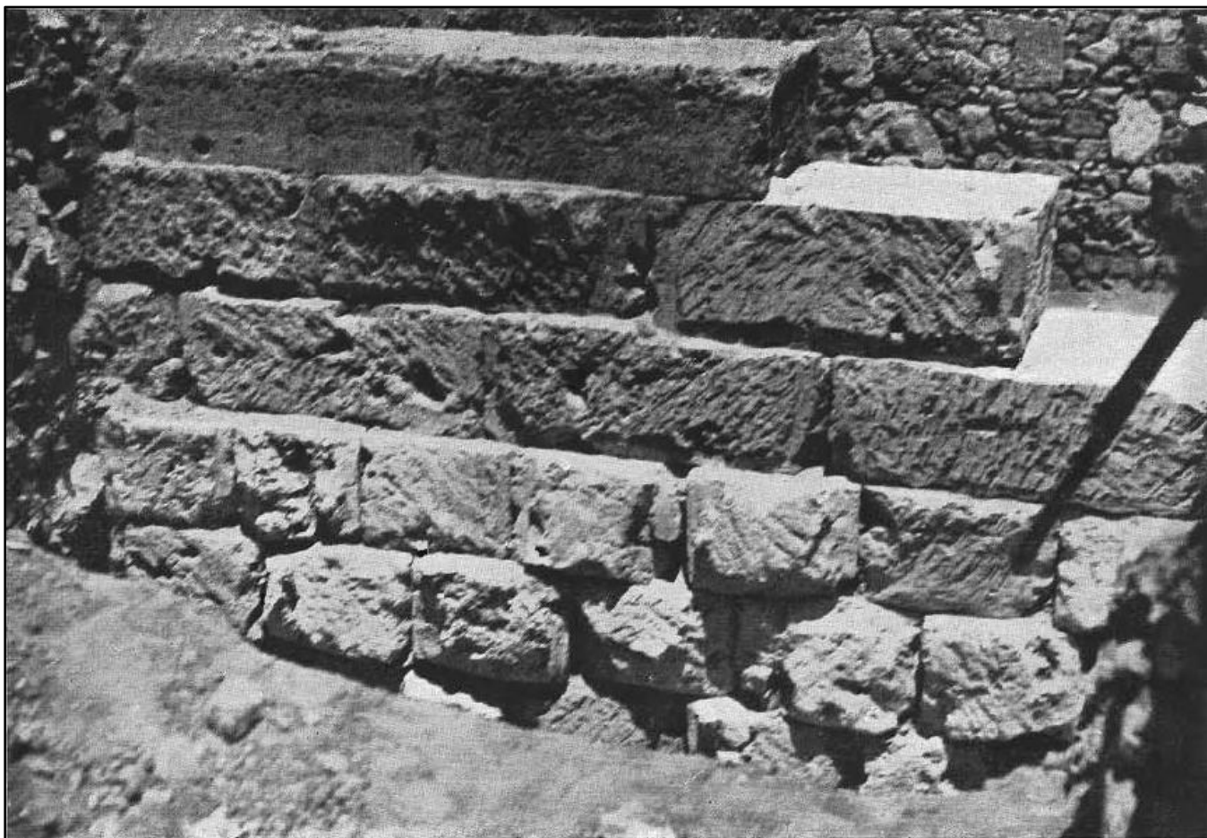
el-Ramleh. Chantier Finney. Construction (No. 17) (Site 120. Adriani 1940a: Pl. VIII, Fig. 1)
