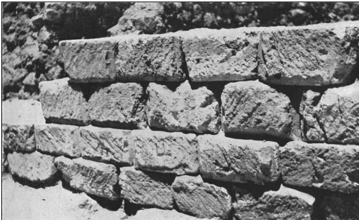
el-Ramleh. Chantier Finney. Construction (No. 1)
