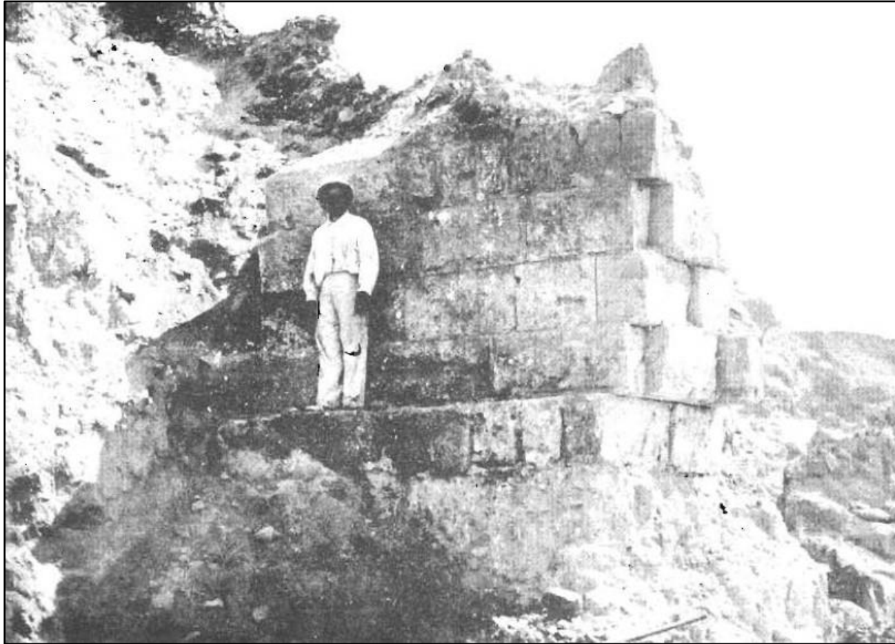
el-Mazarita. Coastal zone, between Cinema Radio and Champollion Street Foundations of nummulithic limestone (Site 133b. Adriani 1934: 66, Fig. 16)
