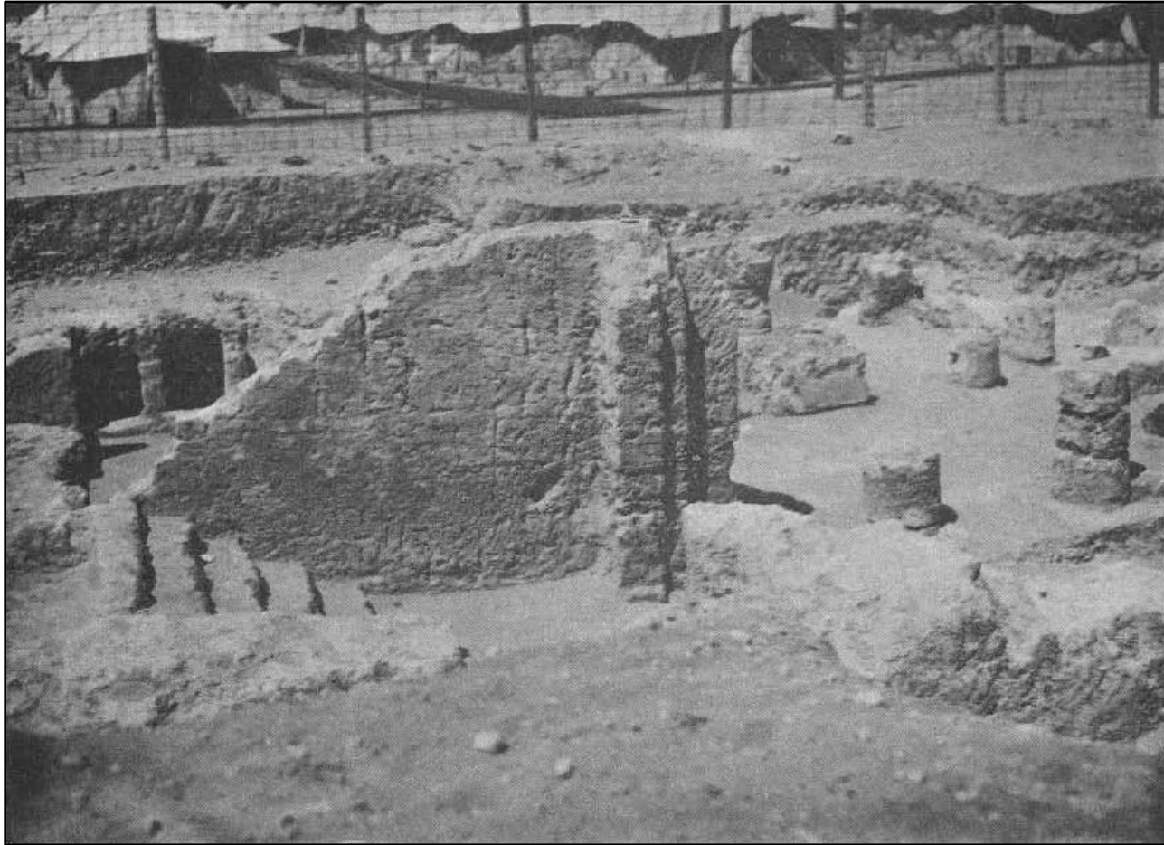
Mustapha Pasha necropolis. Hypogeum (IV). Access-staircase, loculus -chamber, and a peristyle; pre-restoration (Site 160. Adriani 1936: Pl. XXII, Fig. 1)
