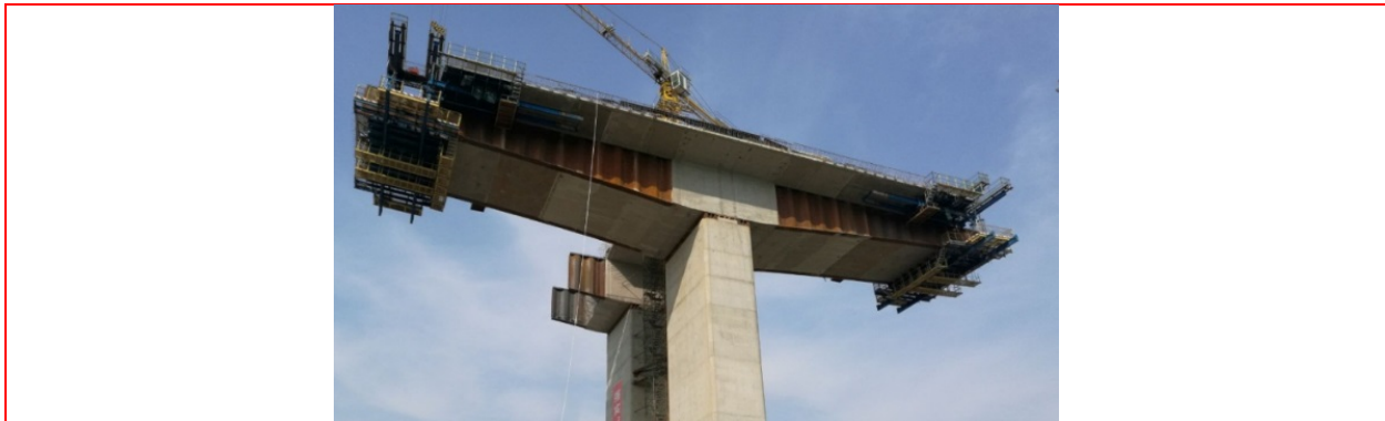
Fig. 8 Composite bridge on-site (China) [48]
