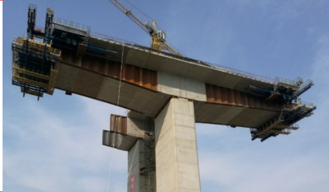
Fig. 4 Composite bridge on site (China) [53]
