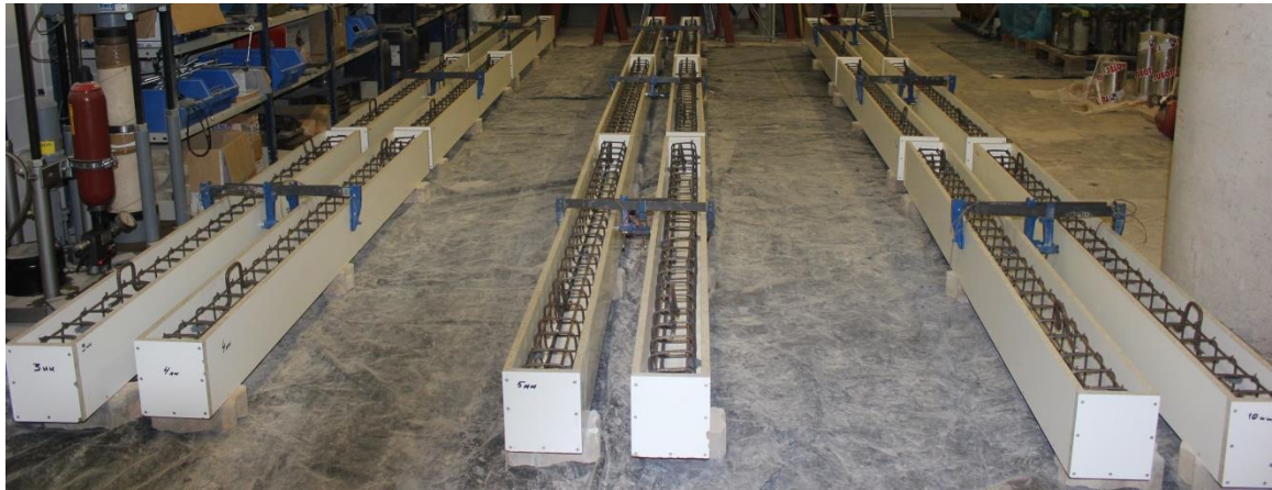
Figure 3.5 Arrangement of beams before casting.
