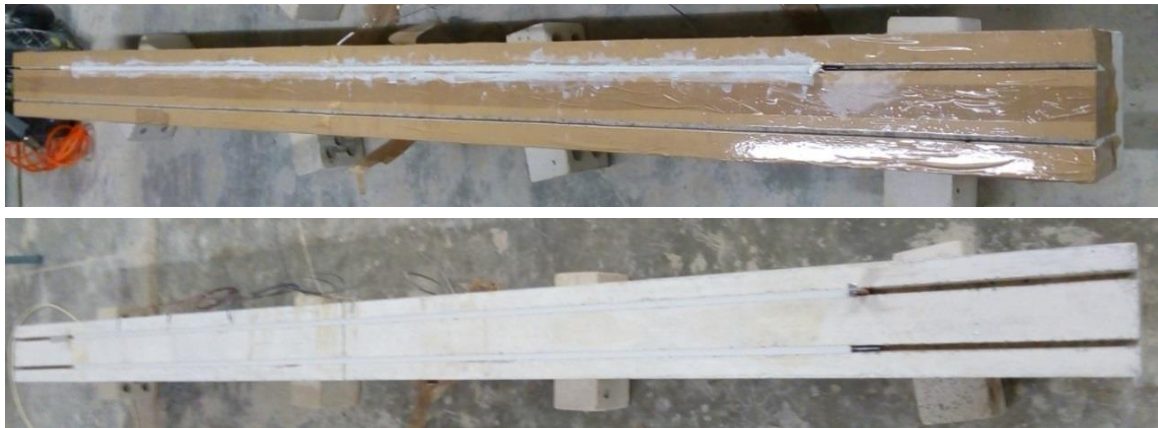
Figure 3.11 Installation of CFRP strips in the grooves.
