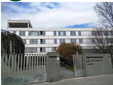
Figure 4-2 Facade of apartment section-View Ronda de Delt
