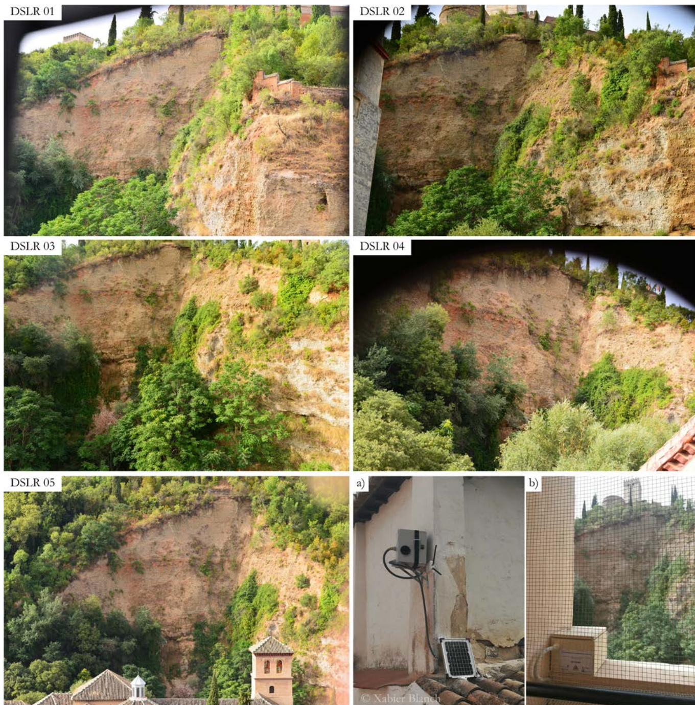
Figure III.8. Images obtained with each photogrammetric system installed in Granada. Images were taken on 12 July 2019 at 09:17h. a) Image of the system installed on the terrace of the Church of San Pedro (DSLR4). The difficulty in installing the system can be seen, as it had to be installed on raised supports. b) System installed in the bell tower of the church (DSLR1), where greater camouflage with the surroundings was required.
