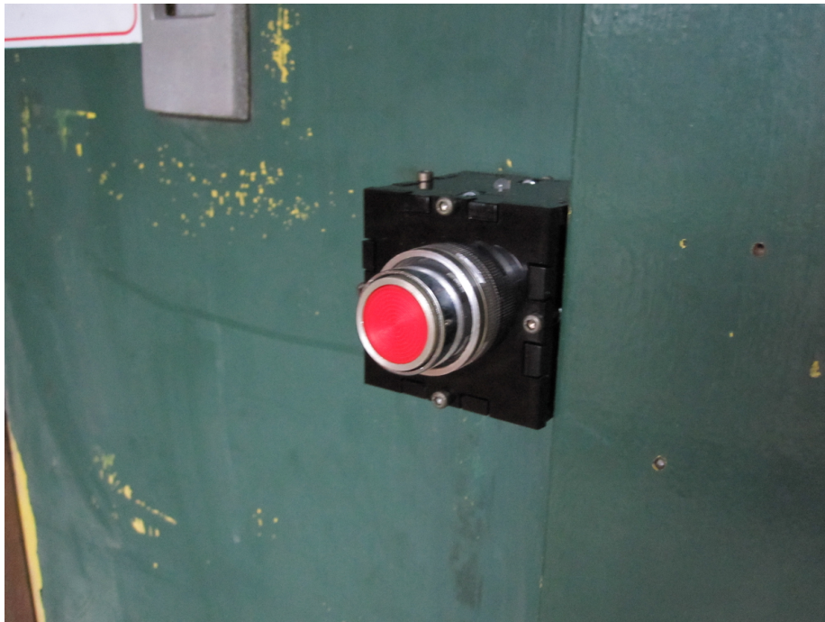
Figure 20: London Hackspace bell installed.
