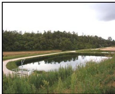
Figure 4.3. Waste stabilization pond WWTP.
