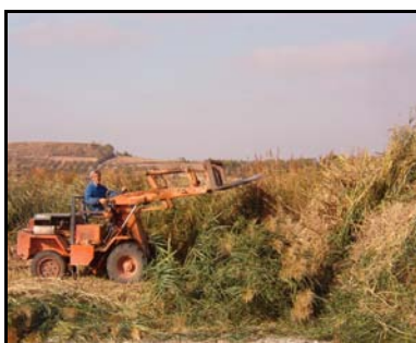
Figure 4.26. Cutting the vegetation of an HSCW using heavy machinery.
