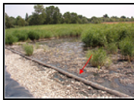
Figure A1.2. Photograph of a corrugated tube for water distribution to the inlet.
