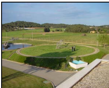
Figure 4.4. Intermittent sand filters WWTP.
