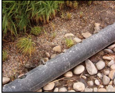
Figure 4.7. Wastewater distribution system through a perforated tube.
