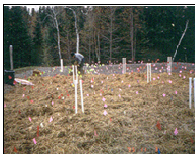
Figure 4.39. Photograph of an HSCW located in Minnesota. The surface is covered with a layer of straw [Source: www.septic.coafes.umn.edu/.../GrandLake.htm ].
