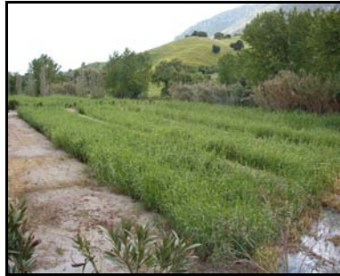
Figure 4.2. Constructed wetland WWTP.
