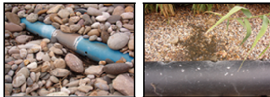
Figure A1.3. Photograph of the different perforated tubes for water distribution to the inlet.
