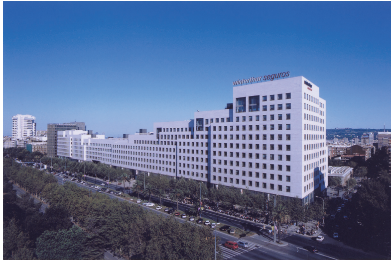
Figura 4.4. C. Climent. Illa Diagonal, Barcelona, 2001
