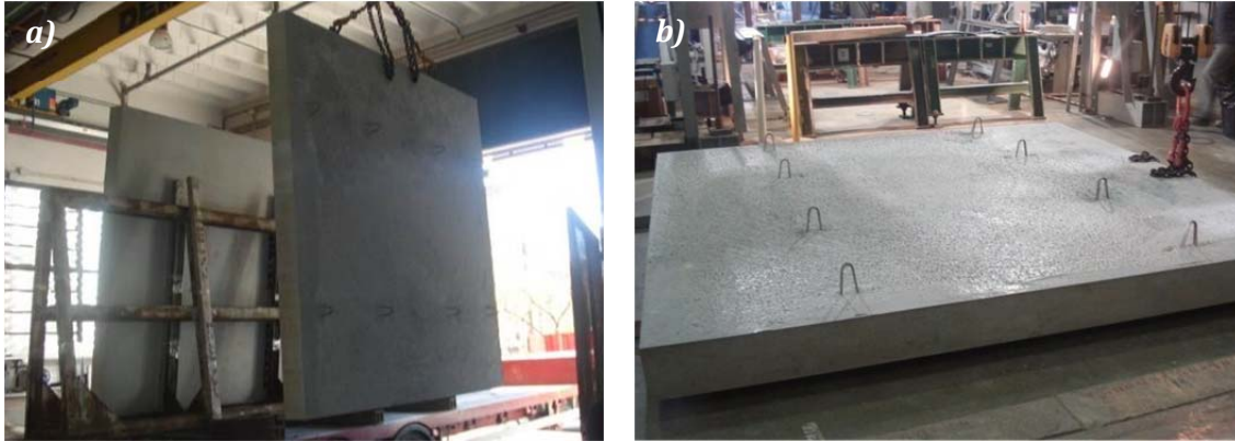
Figure 4.2 Transport of slabs L to the Laboratory of Structure Technology Luis Agulló.
