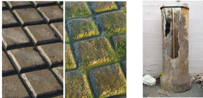
Figure 1.1.- Left: Pavement sailing Club with and without algal colonization. Right: Drain Pipe attacked by *Thiobacillus thiooxidans* ([www.wallisengineering.net](http://www.wallisengineering.net), 2012)
