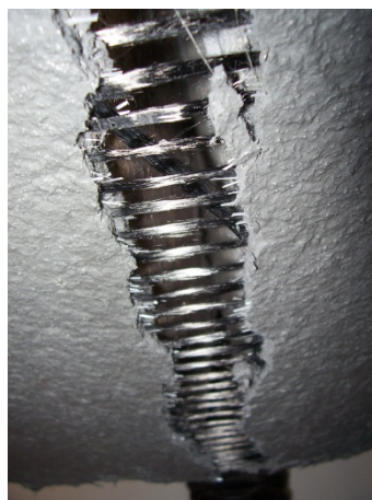
Figure 3.9 Completely open failure crack. TPB tests on sample from the series SP_XMesh
