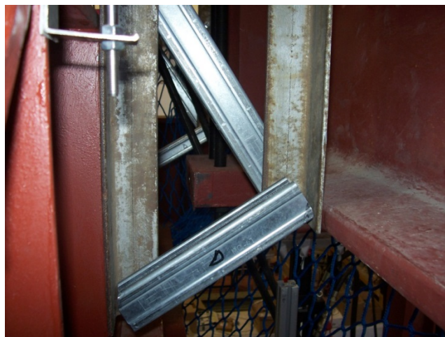
Figure A1. 91 Detail of the steel lattice installed in test setup for walls W#2 to W#5 to control the vertical alignment of the distribution beam during the test.
