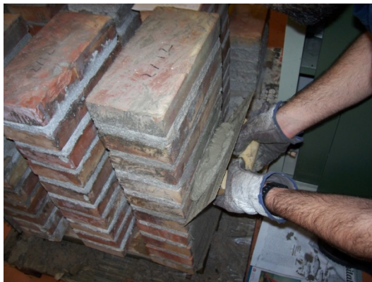
Figure A1. 45. Application of the first mortar layer. Sample M1
