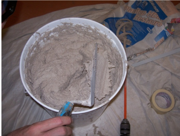
Figure A1. 80 Mortar Planitop HDM Restauro just after being mixed
