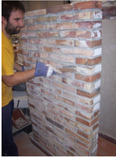
Figure A1. 76 Brushing the masonry surface to remove little mortar irregularities
