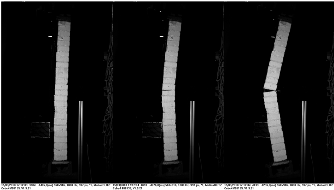
Figure A1. 170 Failure of the wall W#15. Opening of a horizontal joint at mid-height.
