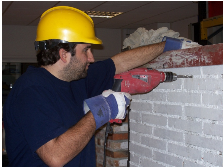
Figure A1. 75 Drilling process of wall W#29
