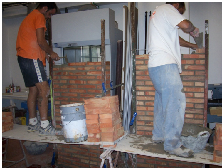
Figure A1. 59 Construction of walls W#2 to W#5
