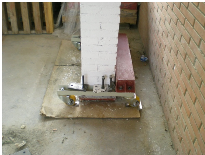
Figure A1. 66 Lifting procedure for wall W#17
