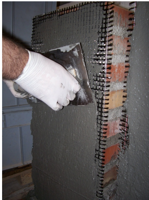
Figure A1. 47. Second mortar layer spreading process for sample X1
