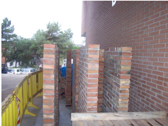
Figure A1. 63 Walls W#10 to W#17
