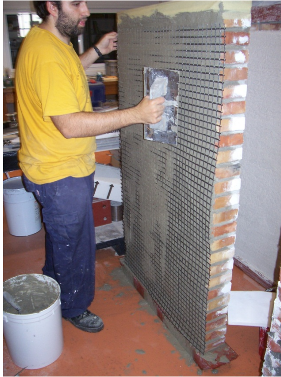
Figure A1. 83 Embedding the glass fibre grid with a trowel
