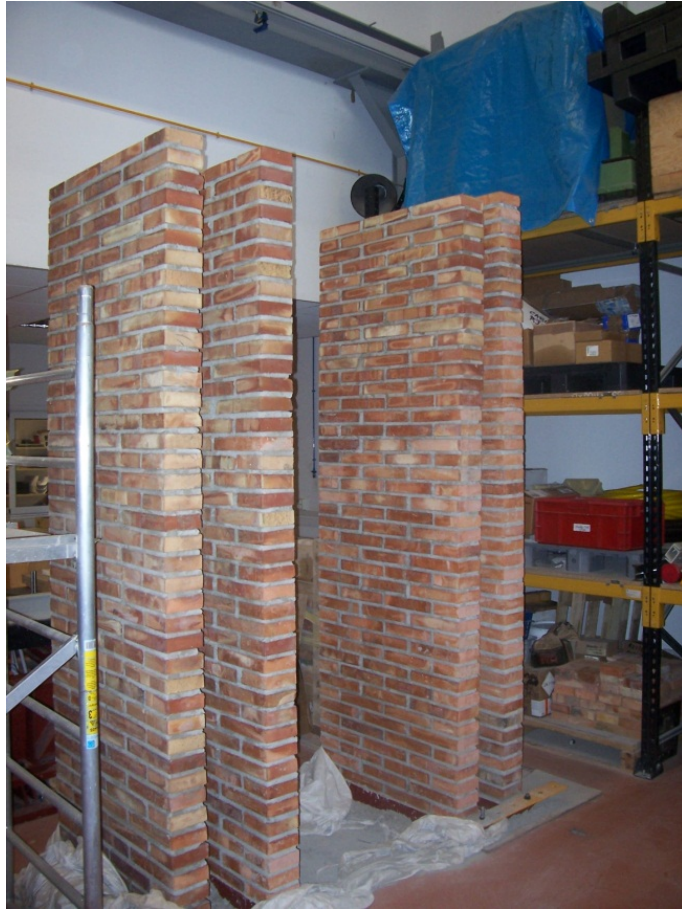
Figure A1. 62 Walls W#6 to W#9
