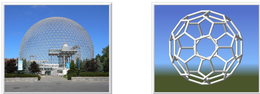
Figure 1.1. Left: Montreal's Biosphere Environmental Museum (Canada) resides inside a Geodesic Dome designed by R. Buckminster Fuller. [2] Right: C_{60} fullerene representation.
