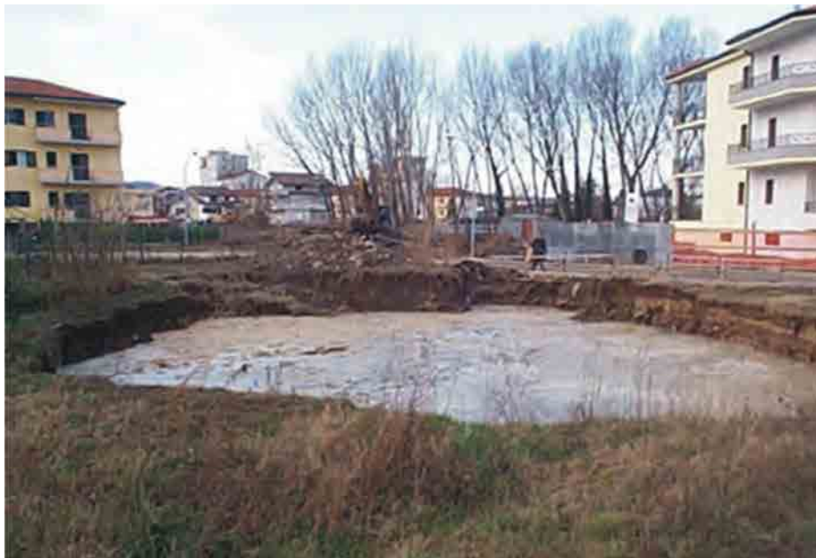
Figure 6.66: Sinkhole occurred in Telese Terme urban area in 2002
