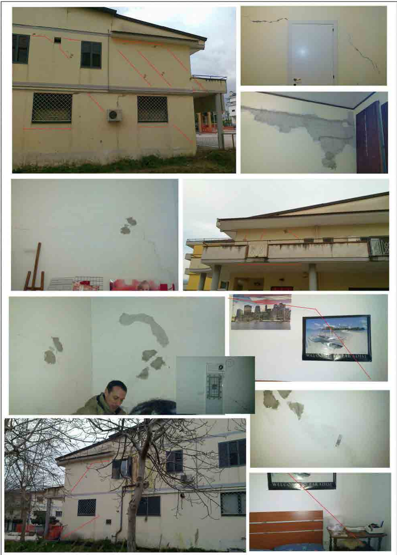
Figure 6.74: Forensic analysis of the building n°2
