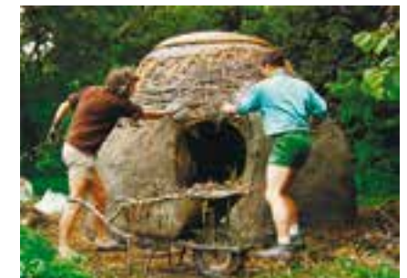
Fig. 404. Cloud Chamber . Willow structure dauded with mud, top and doorway made of reeds. Beelden Buiten, Tiel, Belgium, 1990.
