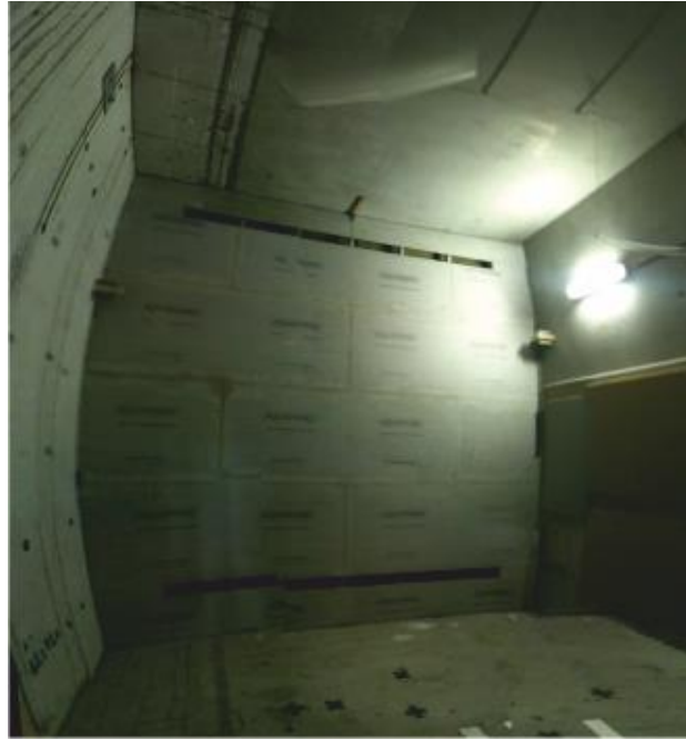
Img.C.7 Prototype installed air cavity 100% ventilated (D1)
