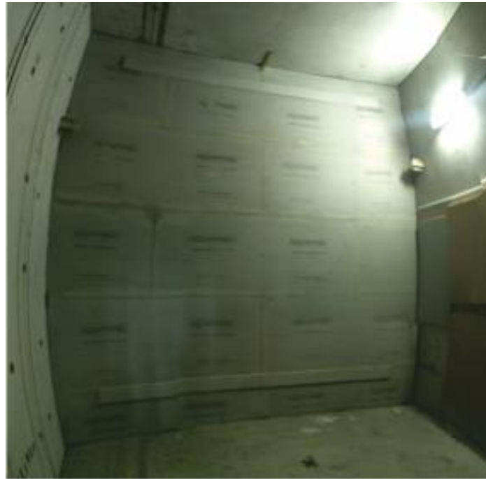
Img.C.9 Prototype installed air cavity 0% ventilated (D1)
