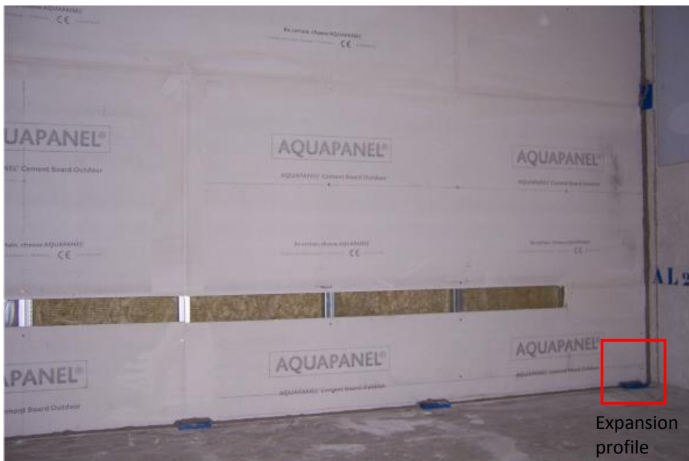
Img.C.4 Detail installed prototype (D1)
