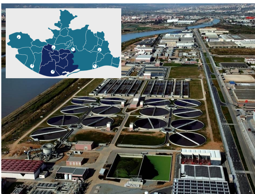
Figure 4.2. Aerial view of Baix Llobregat WWTP (Barcelona, Spain).
