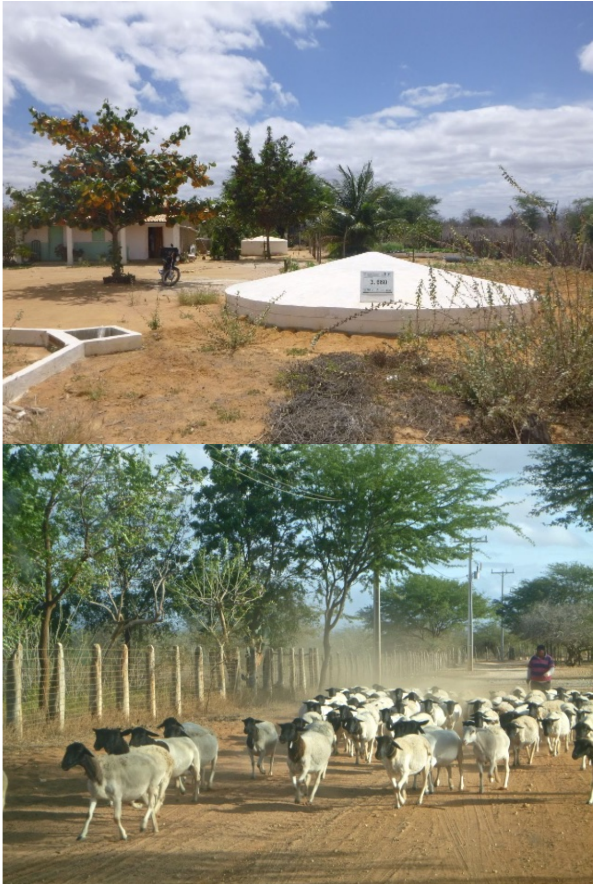
Picture 3. Program “1 milhão de cisternas”, reservoirs for rainwater harvesting and goats, at the Salitre River Basin in Bahia, Brasil.
