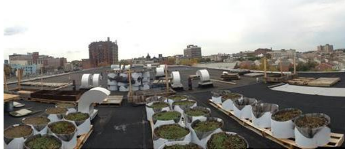
Figure 1.9. Rooftop garden of Cloud 9 (Philadelphia, USA).
