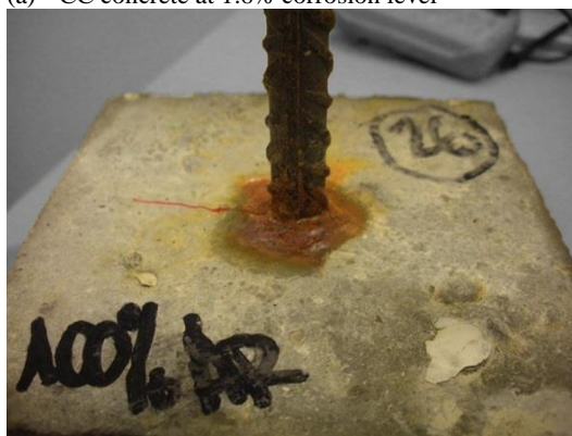
(c) RAC-100 concrete at 1.6% corrosion level
