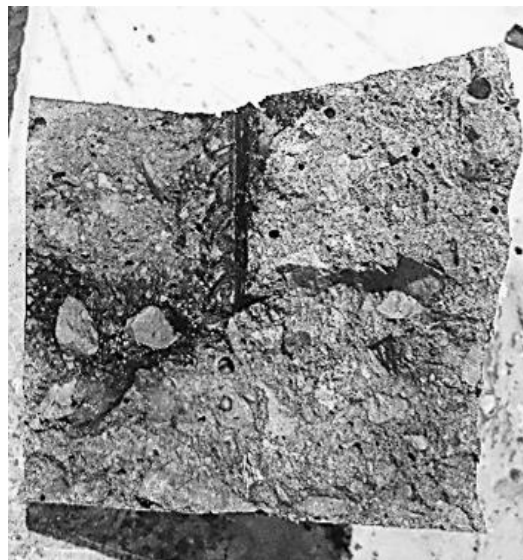
Figure IV-29. Internal damage cracking for RAC-100
