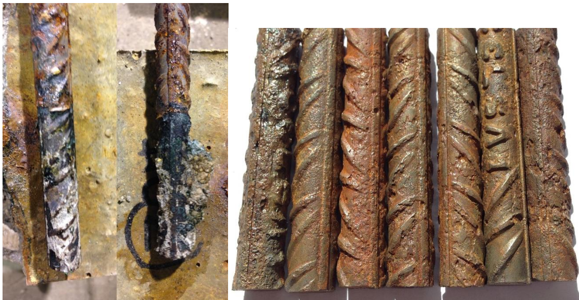
Figure IV-26. Steel bar specimens before and after cleaning procedure
