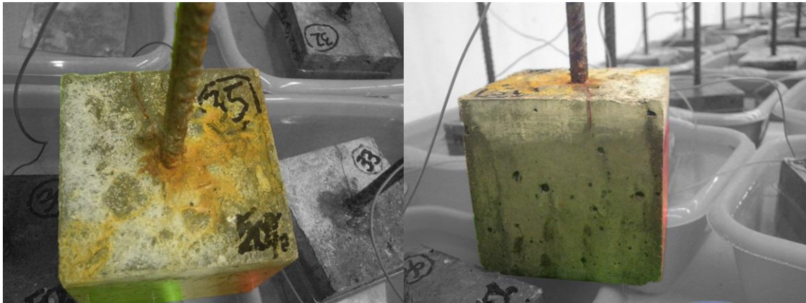
Figure IV-28. Surface cracking of RAC-50 at 5.75% of corrosion level
