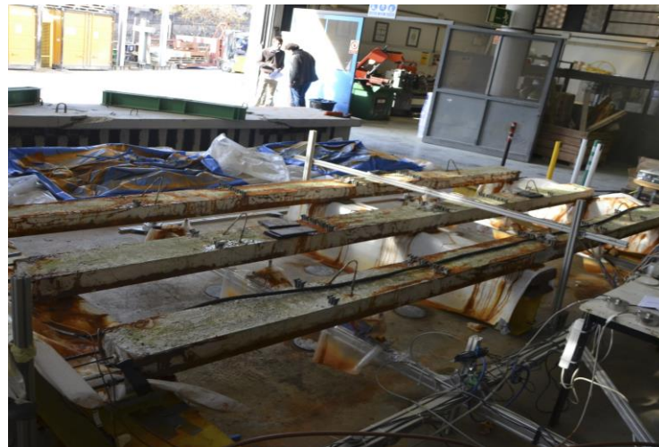
Figure IV-2. Statically indeterminate corroded beams and extracted steel reinforcement
