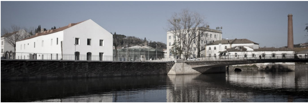
Figure 4.19. Casa dos Cubos, View of the building, after the intervention, and its surroundings
