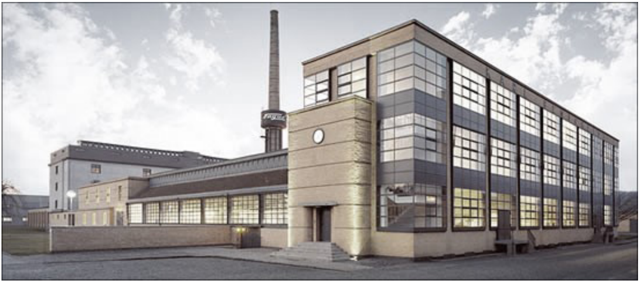
Figure 3.8. Fagus Werk, Alfeld on the Leine, Germany (Source: Fagus Factory, 2014)
