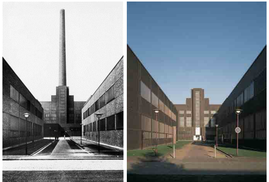
Figure 3.27. German Design Centre, Essen, Germany (Source: Foster + Partners, 1997)
