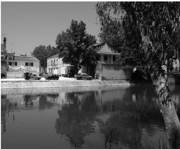
Figure 4.13. Casa dos Cubos, Storehouse before the intervention (Source: courtesy of Embaixada Arquitectura)
