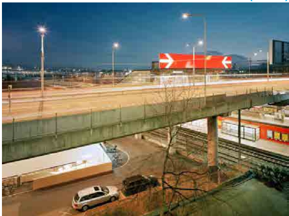
IC219: Hardbrücke Railway Station Upgrading, 2004-07
