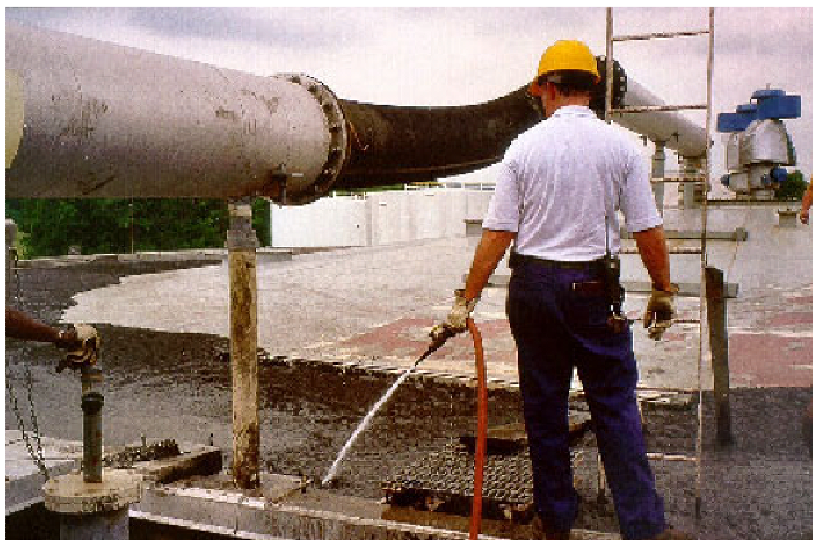
Figure 2.7. Biological foaming in an anaerobic digester (Massart et al. , 2006).
