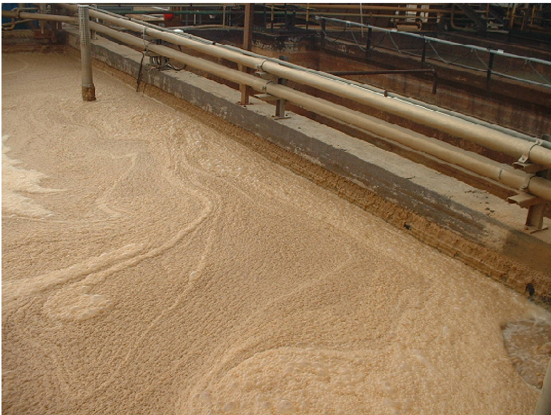
Figure 2.6. Biological foaming in a biological reactor.
