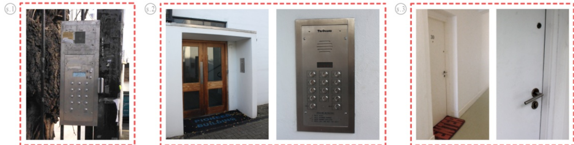
Three different security filters that the user finds in the main Pioneer Health Centre itinerary while trying to get to his flat. From left to right, enclosure door with pass code (s.1), building's main door with another pass code (s.2) and flat's door opened with a set of keys (s.3).
