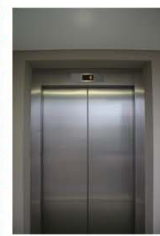
06 Lift room Waiting for the lift
