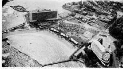
HOTEL BEING BUILT ALONG THE HISTORIC POINT LINE, DESIGNED BY OLD SAN DOMINGO CASTLE (UPPER LEFT).
