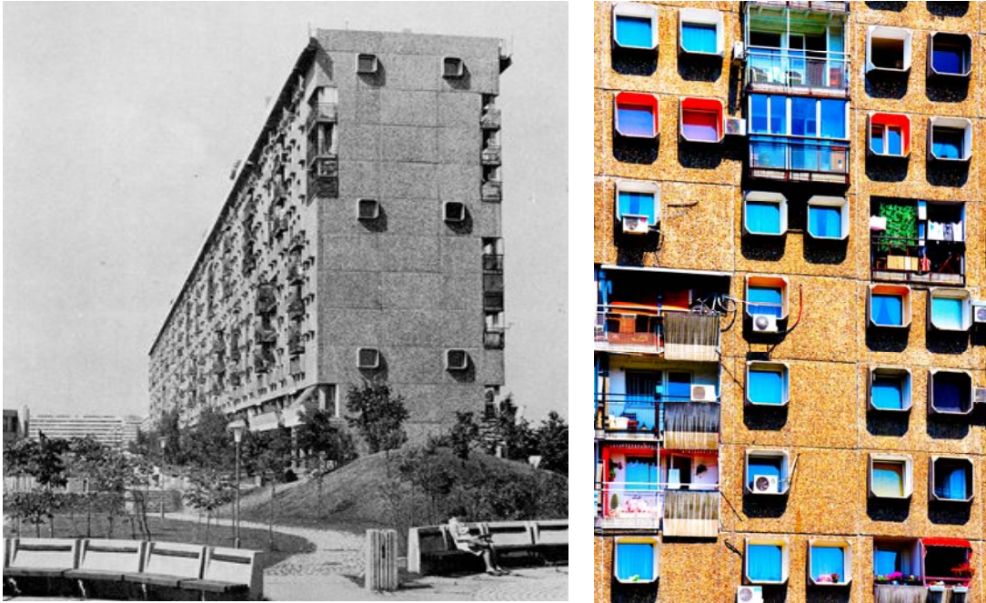
Figure 22: Block No.28 - TV buildings (IMS load-bearing construction system with "Keramzit" façade panels)
