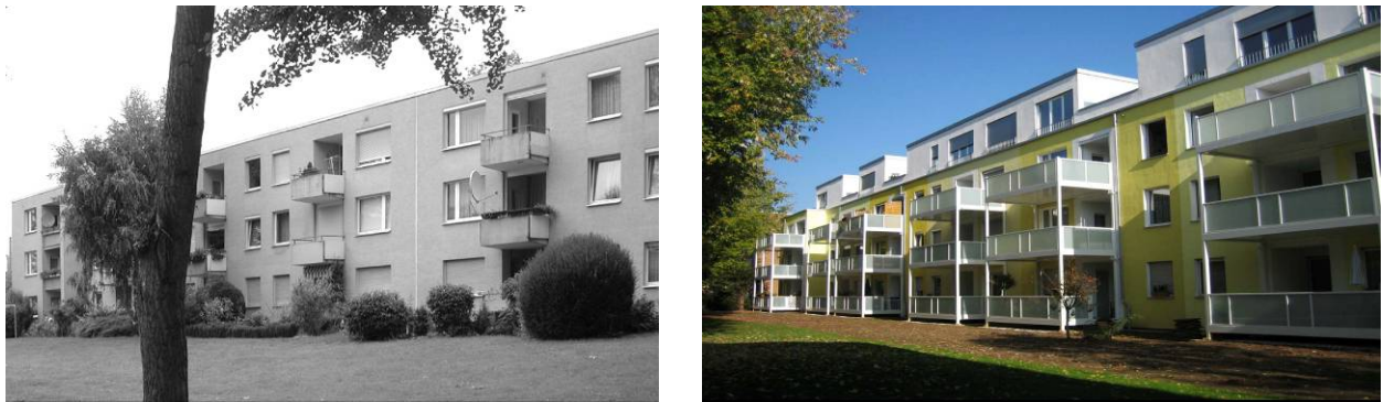
Figure 124: Annex of attics on the top of the flat roofs: Three-storey block in Praunheim, a district of Frankfurt am Main(T S B Consulting, 2007), see: Appendix - Refurbishment scenarios for post-war housing in Europe: State-of-the-art
