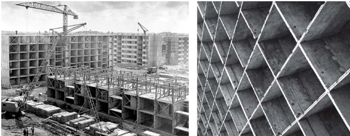
Figure 14:Yugomont YU61 large panel system - construction work in progress
