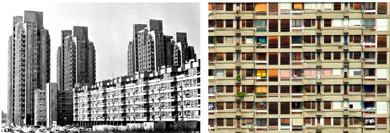
Figure 21: Block No.23 - Variety of prefabricated components applied in the façade
