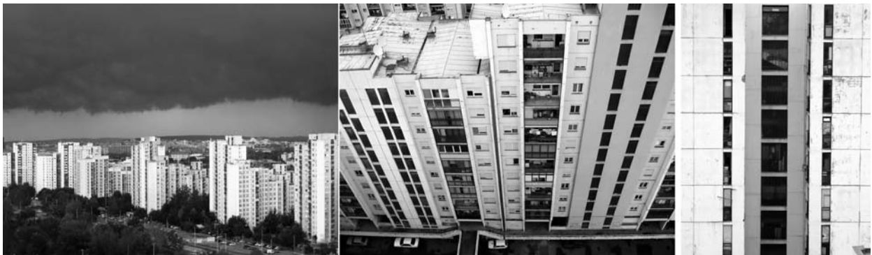
Figure 26: Block No. 64: Rad-Balency huge panel industrialized system (fotos by Goran Jovanovic)
