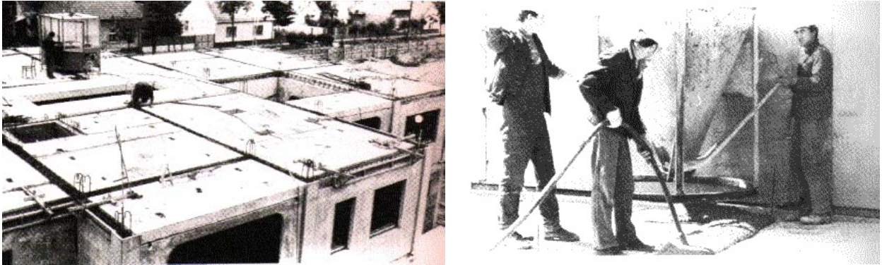
Figure 12: Montastan building assembly: construction in progress 4
