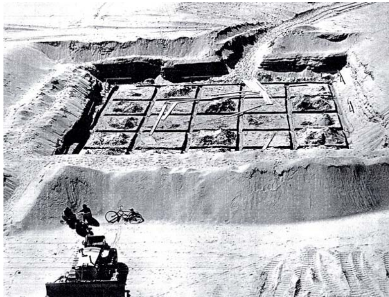
Figure 55: Reinforced concrete strip foundation
