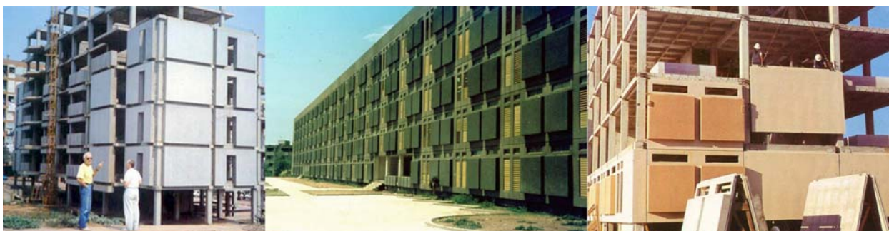
Figure 16: IMS housing in Cuba and Angola: building assembly process
