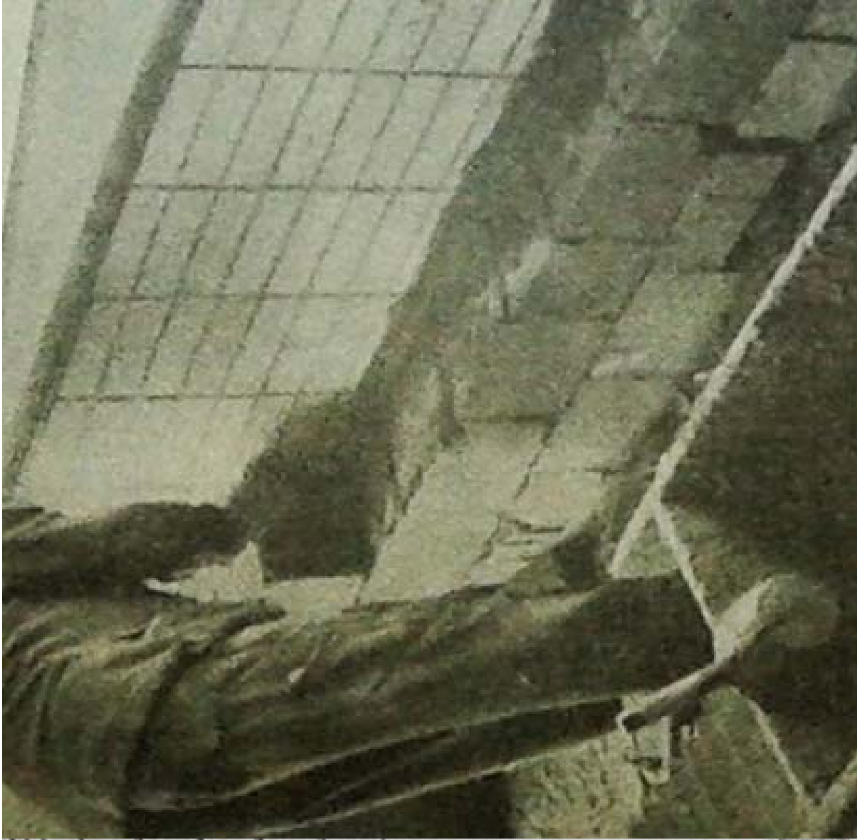
Figure: Combination of conventional and prefabricated systems in façade construction (Block No.21-Industrialized concrete parapet (6 cm + ceramic tiles), conventional brick parapet from the inside)
