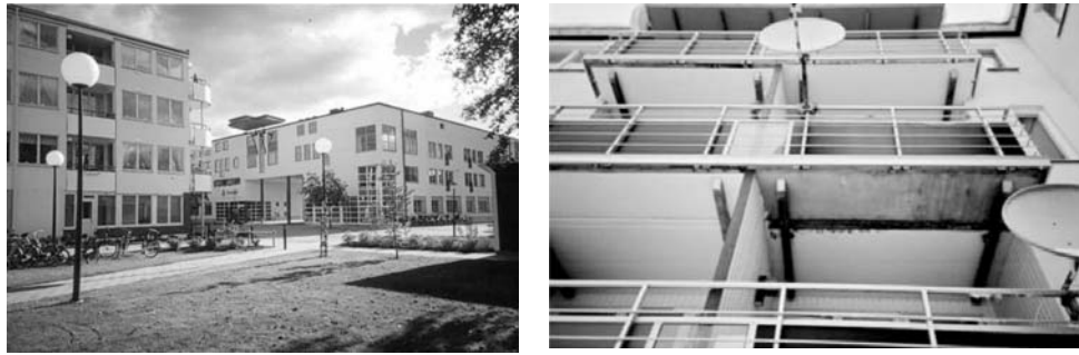
Figure 26: Construction of the balcony extension
