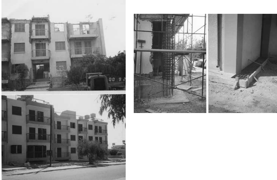
Figure 9: During the renovation and after the completion of the works
