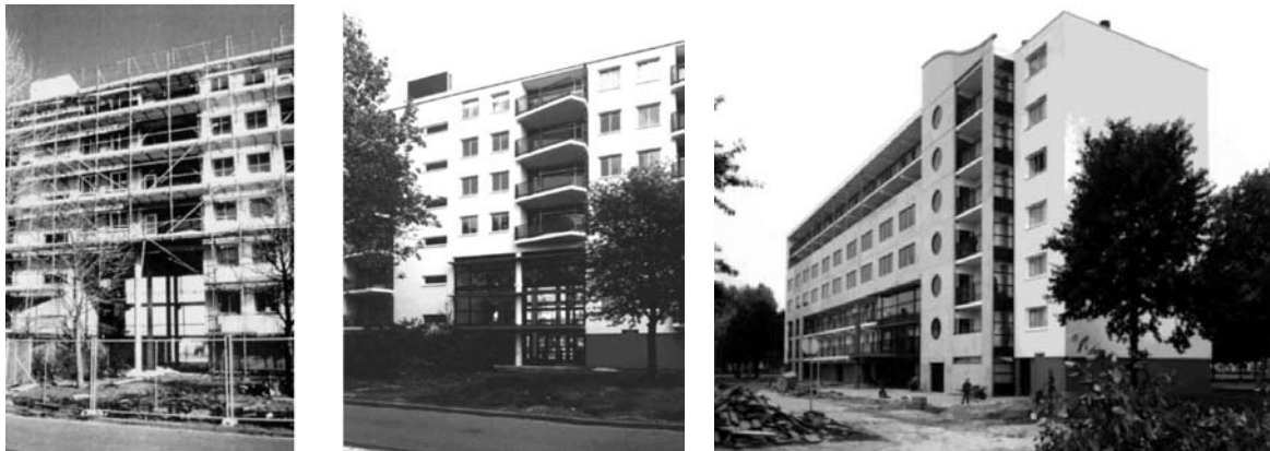
Figure 24: Building model before and after façade refurbishment
