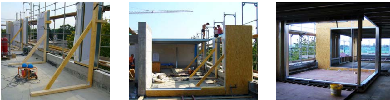
Figure 31: Attic construction in progress
