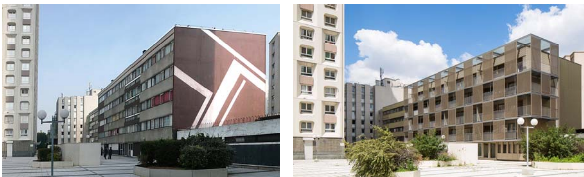
Figure 16: Building model before and after façade refurbishment
