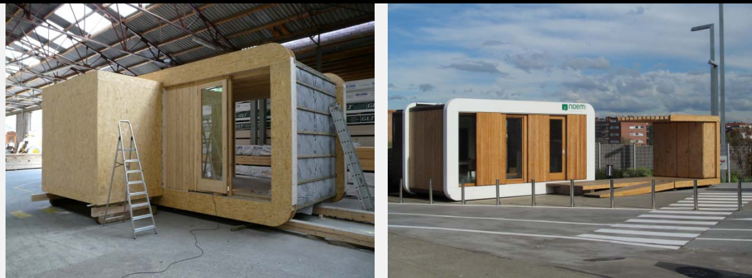
Figure 44. This is a modular system of wood with walls constructed from frames (A-4). Figure 45. The module positioned on-site (A-4).
