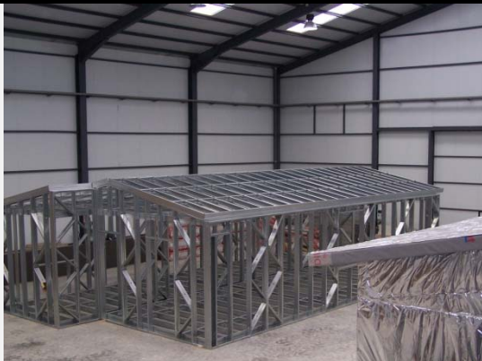
Figure 40. This is a room module with steel frame walls. Figure 41. A house constructed using this system (A-20).
