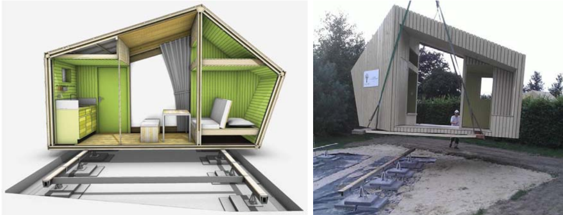
Figure 17. The building is a wooden bungalow with concrete footings made from demolition waste [Moonen and Hermans, 2013]. Figure 18. A crane is used to position the bungalow over its foundation.
