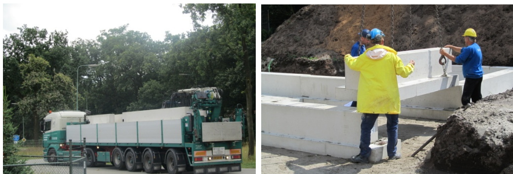
Figure 154 and 155. Transport and positioning of precast continuous footings.
