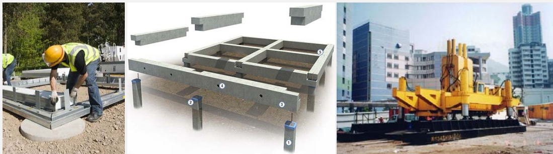
Figure 62. Pile caps and the floor can be precast. http://www.roger-bullivant.co.uk/images/photos/system1.jpg Figure 63. Precast concrete piles with precast ground beams. http://charconcs.com/sites/default/files/editor/charconCS-FASTBEAM-main-section_01.jpg Figure 64. Multifunctional hydraulic static pile driver. http://img.isp.org.cn/nimg/04/95/1bd832dc4f9904aaef37f431ff6a-200x200-1/zyc900b_b_multifunctional_hydraulic_static_pile_driver.jpg
