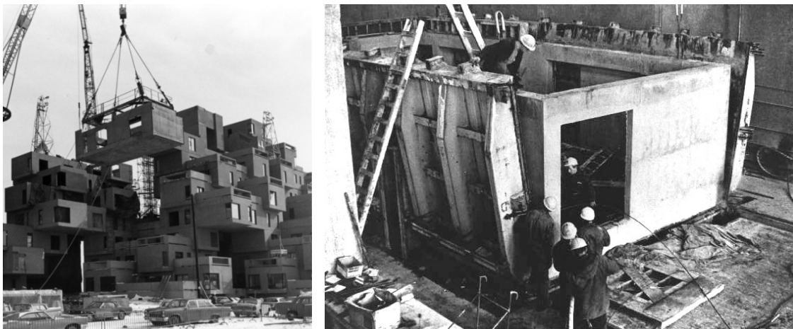
Figure 30. Habitat '67, a room module designed by Moshe Safdie and built for Expo 67 in Canada. The modules were put in place using a crane. https://s-media-cache-ak0.pinimg.com/236x/b4/1c/64/b41c64707e719e56c09351c40552ae7b.jpg Figure 31. Construction of a module in the factory. http://cac.mcgill.ca/safdie/habitat/constructionPhoto.php?stage=1
