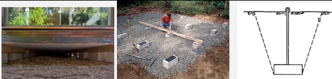
Figure 102. Block foundation for a studio. http://www.settstudio.com/ Figure 103. Block foundation for a backyard shed. http://www.finehomebuilding.com/how-to/articles/firm-foundation-backyard-shed.aspx Figure 104. They can also prevent uplift [Kovacs and Yokel, 2014].
