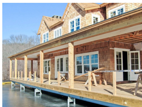
Figure 152. Screw micropiles can be a good solution when there is a slope. Figure 153. Or when they are in contact with water. http://www.archiexpo.es/prod/techno-pieux-inc/product-61493-992253.html
