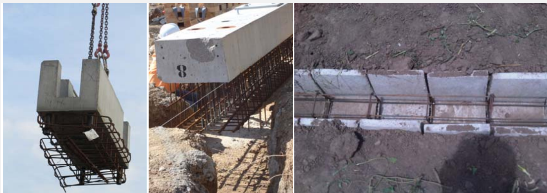
Figure 99. Semi-prefabricated strip footing for a panel modular house. Figure 100. Semi-prefabricated precast ground beam with piles. Figure 101. Semi-prefabricated strip footing made up of parts.
