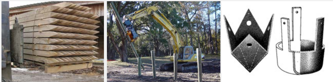
Figure 65. Storage of timber piles. http://sachsen-anhalt-nebra.annoncen.org/export/handwerk-20120614121341.png Figure 66. Timber pile driver. http://www.myrickmarine.com/project/house-timber-pile-foundation/ Figure 67. Protective attachments at the pile tip and pile head can be used to prevent splitting and brooming of the pile. https://www.pilebuckinternational.com/wp-content/uploads/2013/11/timberpts1a.jpg
