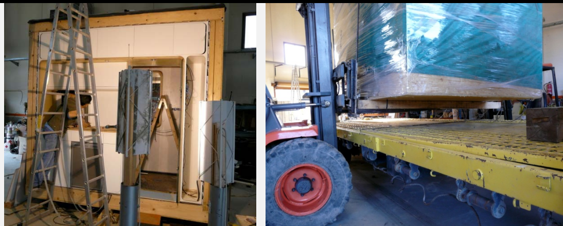
Figure 48. Modules are complete when they leave the factory. This module includes the kitchen, bathroom, plumbing and wiring (A-6). Figure 49. The modules are light and easy to handle and transport. They can be packaged so that they do not get damaged (A-6).
