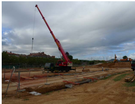
Figure 137. Placing of precast pads. Figure 138. Crane to place precast pads.
