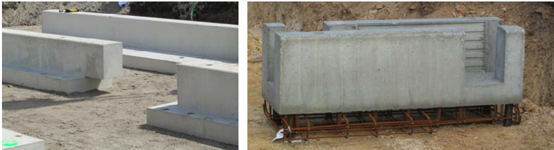
Figure 56. A precast strip footing is a prefabricated foundation. Once it is on-site, it must be assembled and the joints are sealed. Figure 57. A semi-prefabricated strip footing is a foundation that must be finished on-site. Once it is on-site, concrete must be added under the element.
