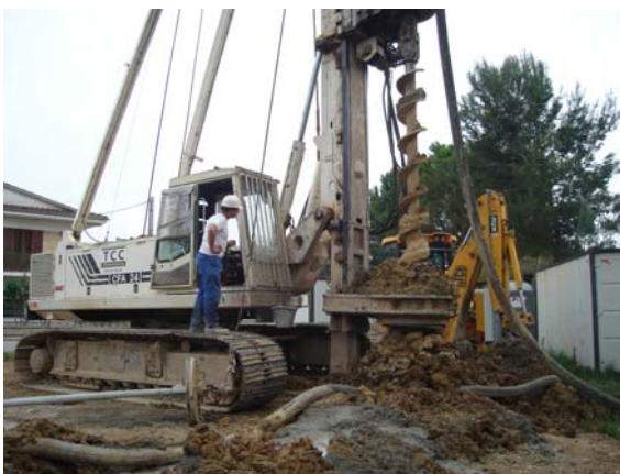
Figure 124. Construction of continuous flight auger piles. Figure 125. Concrete pump and truck mixer.
