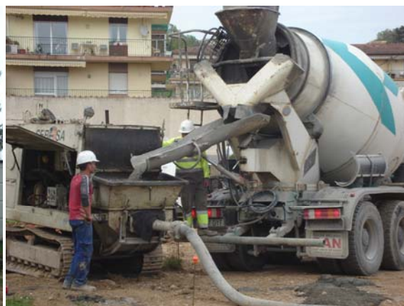
Figure 124. Construction of continuous flight auger piles. Figure 125. Concrete pump and truck mixer.
