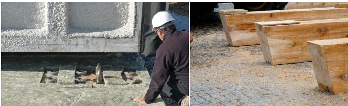
Figure 34. Modules on connectors (A1-16). Figure 35. Modules on wooden beams (A1-4).
