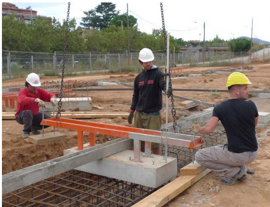
Figure 137. Placing of precast pads. Figure 138. Crane to place precast pads.
