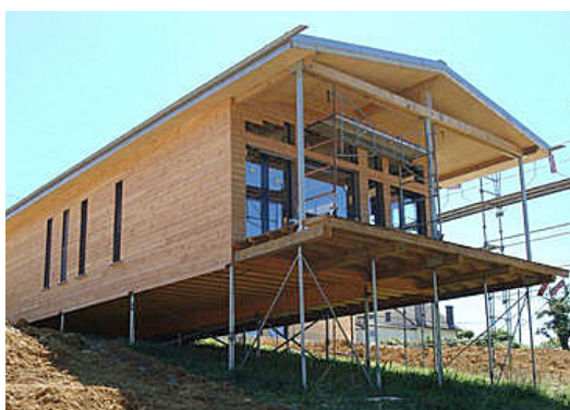
Figure 152. Screw micropiles can be a good solution when there is a slope. Figure 153. Or when they are in contact with water. http://www.archiexpo.es/prod/techno-pieux-inc/product-61493-992253.html
