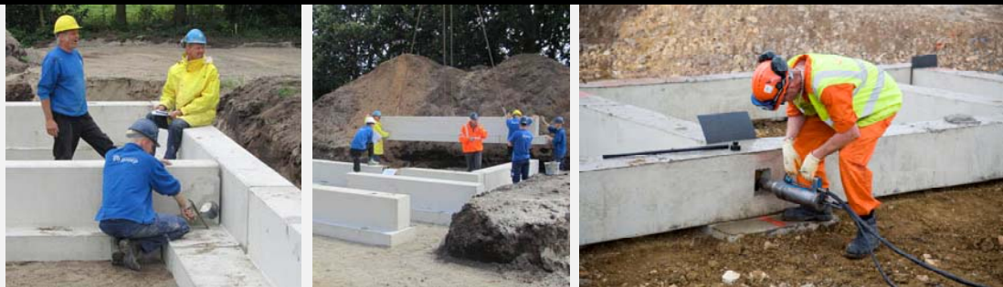
Figure 96. A precast strip footing foundation. Joints must be sealed with mortar. Figure 97. They are put in place using a crane. Figure 98. They can be post-tensioned. http://www.van-elle.co.uk/services/Smartfoot/
