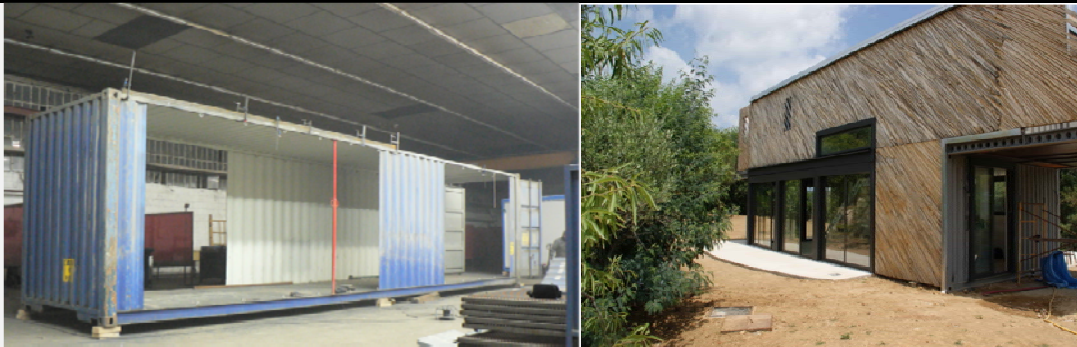
Figure 42. Various shipping containers have been adapted to make this house (A-26). Figure 43. The finished house whose structure is comprised of shipping containers (A-26).
