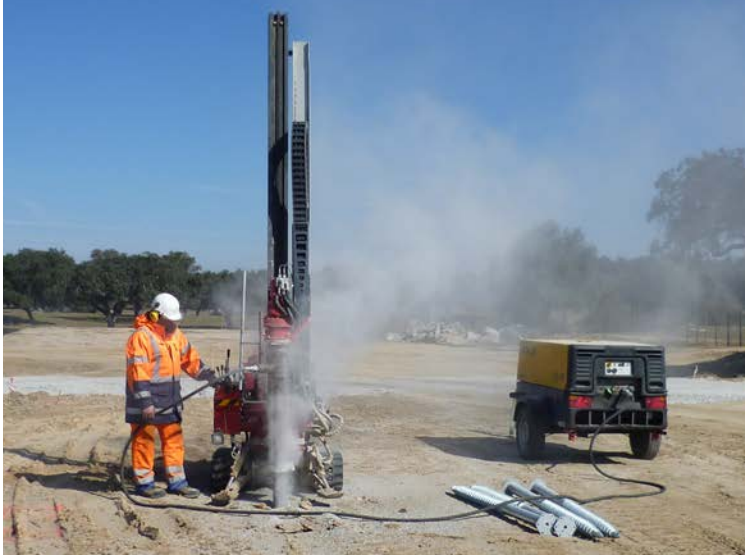
Figure 1. Driving the screw pile into the ground.
