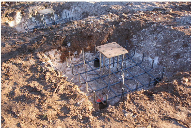
Figure 4. Isolated footing reinforcement before concreting.
