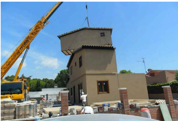
Figure 4. Positioning a module.
