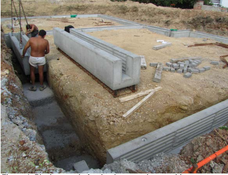
Figure 1. Placing a strip footing by crane into position.
