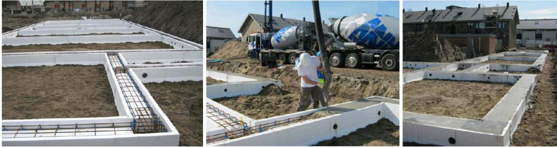
Figure 1. Ground beams before concreting. Figures 2 and 3. Concreting the foundation.
