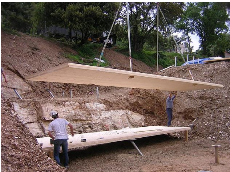
Figure 1. Screw pile foundation for a timber panel house.
