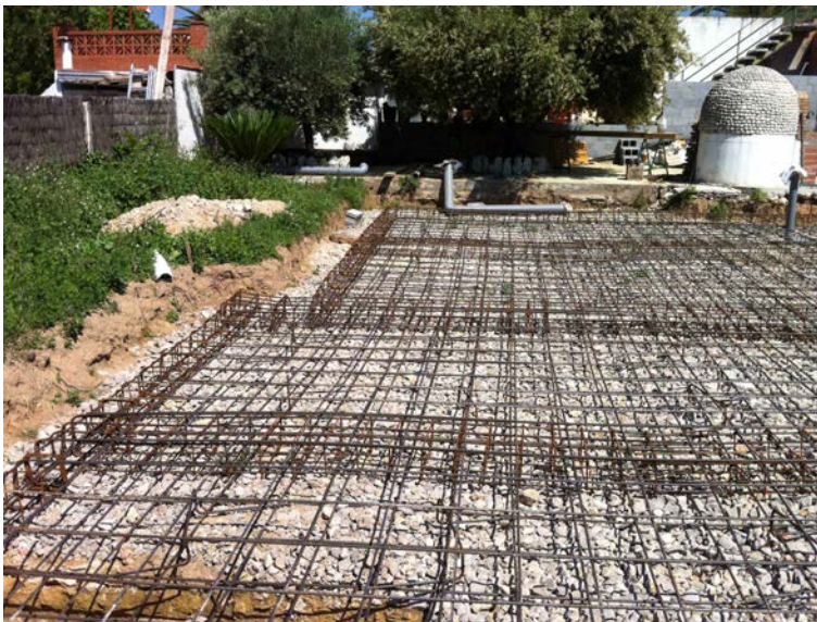
Figure 4. Ground slab reinforcement over a base course.
