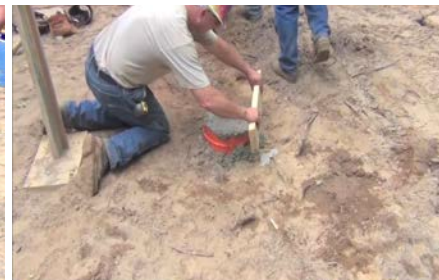
Figure 7. The framework is filled with concrete and pressed. Figure 8. And it is flattened with a board. 2
