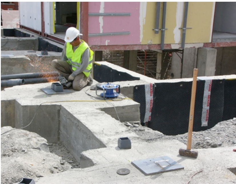
Figure 5. The cutting of offset connector bolts with an angle grinder.
