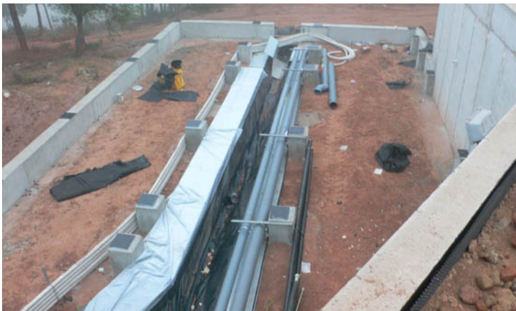
Figure 4. The foundation is prepared to place the modules.
