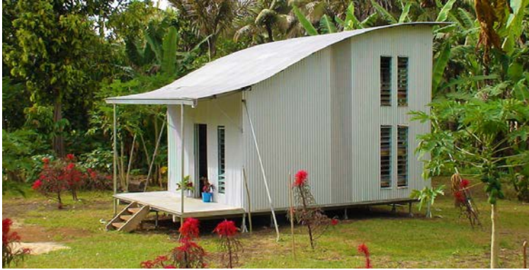
Figure 1. Micropiles house foundation. 1
