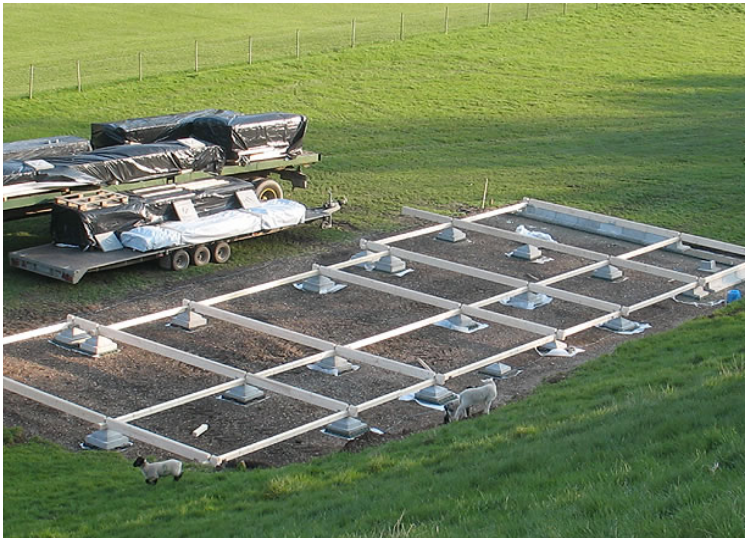
Figure 1. Concrete pad foundation. 2
