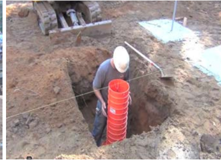
Figure 1. Digging out holes. Figure 2. Land-levelling holes with a layer of gravel of 5 cm. The framework is assembled, placed and leveled in the hole.
