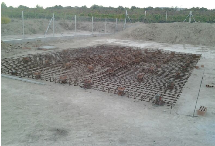
Figure 4. Ground slab reinforcement.
