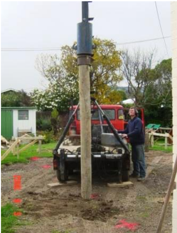
Figure 1. Timber pile driving. 2
