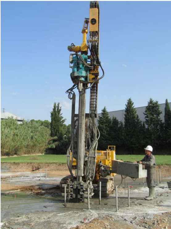
Figure 1. Drilling and injecting grout through the hollow reinforcing tendon.
