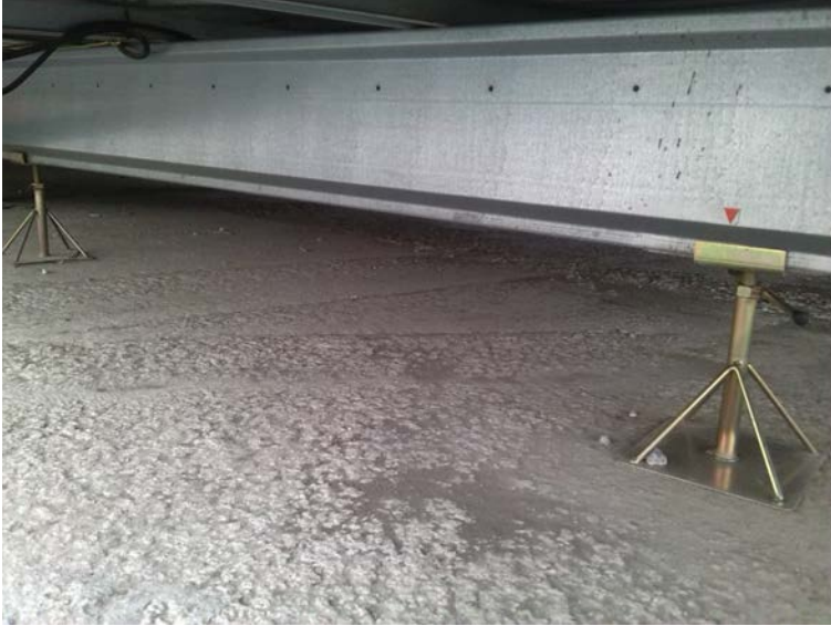
Figure 3. Metal piers support the mobile home over the cast-in-place ground slab.
