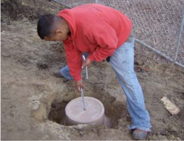
Figure 1. Each base can be maneuvered by hand into position. Lifting inserts allow contractors to easily move these pieces around by hand. 2
