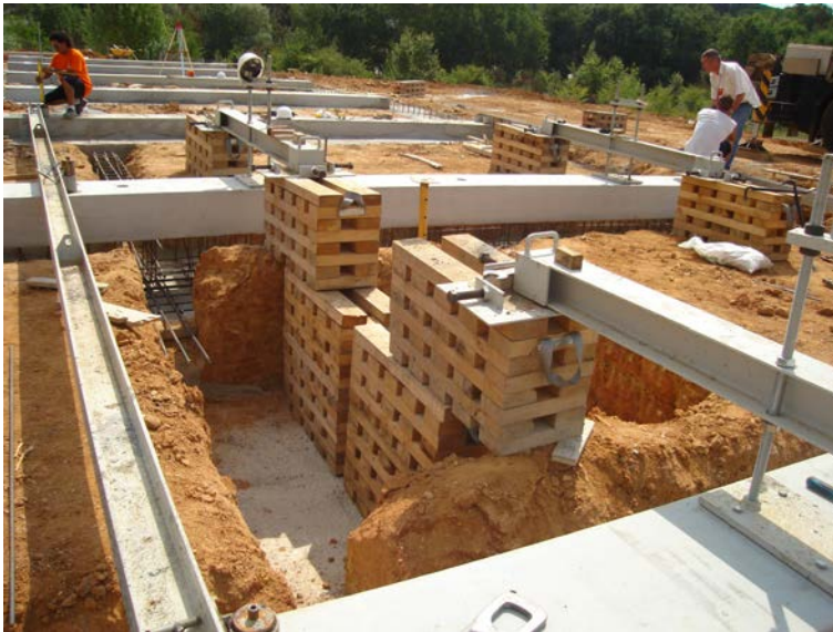
Figure 4. Mechanisms to place prefabricated beams at the right position.
