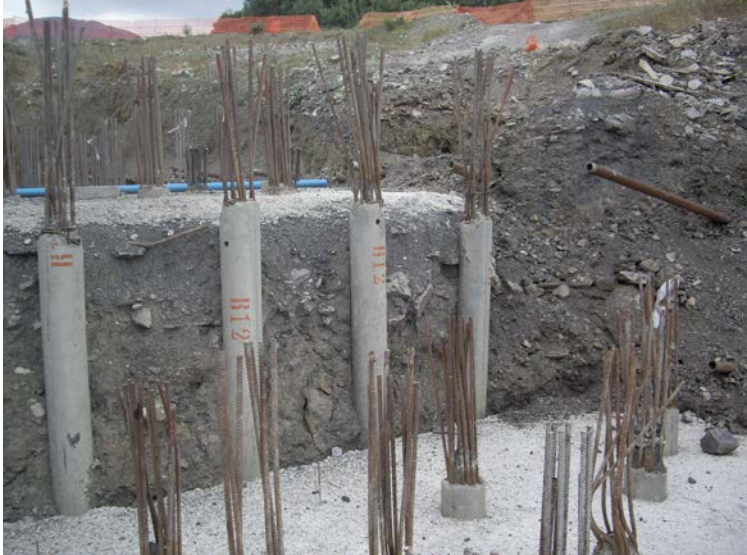
Figure 1. Precast concrete micropiles.
