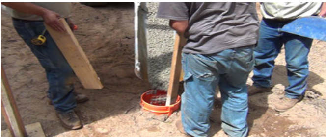
Figure 7. The framework is filled with concrete and pressed. Figure 8. And it is flattened with a board. 2
