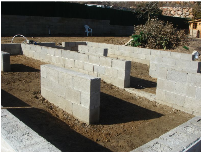
Figure 4. Concrete block walls were built over the foundation.
