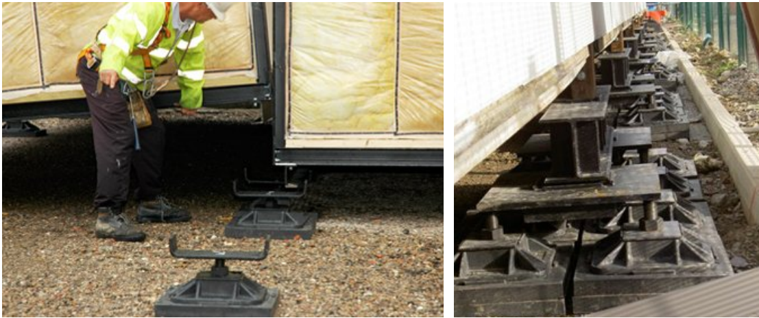
Figure 1. Plastic pads in a modular building. 2 Figure 2. Four pads combined. 3
