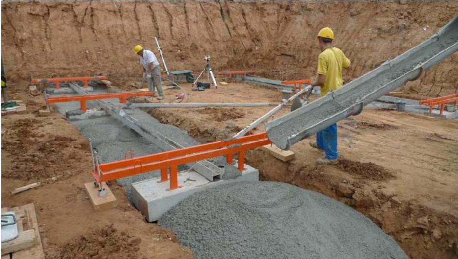
Figure 5. Mechanisms to position precast concrete pads over continuous footings.
