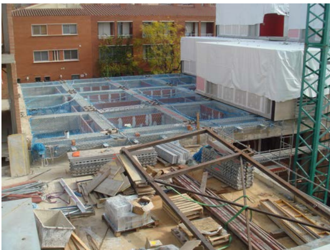
Figure 4. This metal template helped to position module connectors to the right position.
