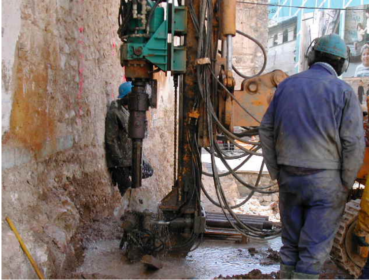
Figure 1.Placing the tubular reinforcement.
