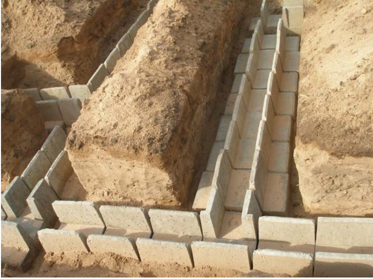
Figure 1. Precast strip footing foundation.
