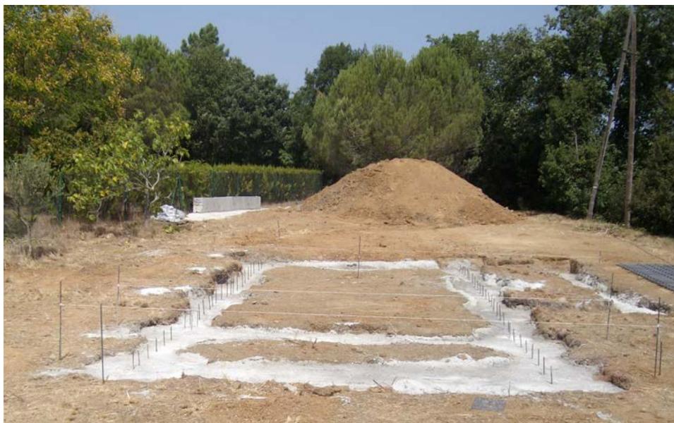
Figure 4. Cast-in-place strip footings and tie beams.
