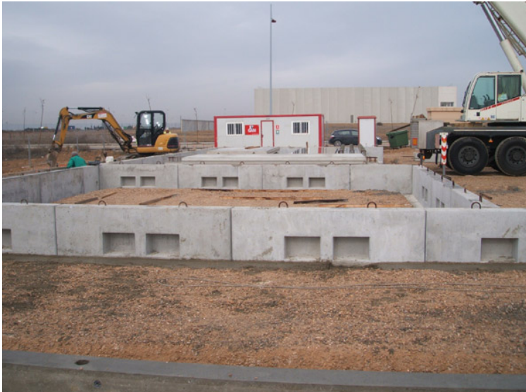
Figure 1. Precast strip footing foundation. 2
