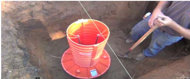
Figure 3. Rebars are hold in the plastic framework. Figure 4. The hole is filled with backfill.
