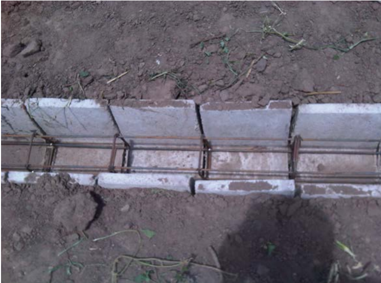
Figure 2. Precast strip footing foundation with rebar.
