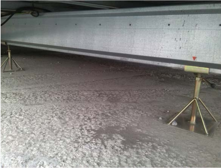
Figure 1. Metal pier over a concrete ground slab.
