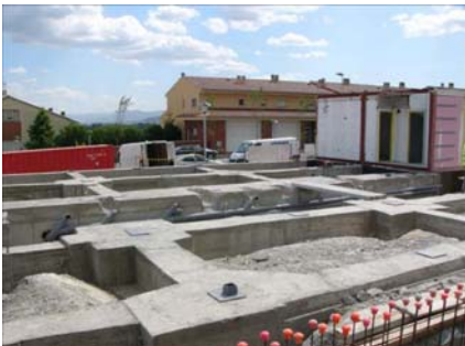
Cast-in-place foundation
