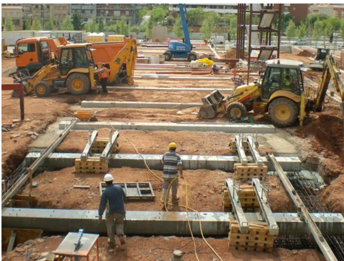
Figure 6. Mechanisms to place prefabricated semi-beams.
