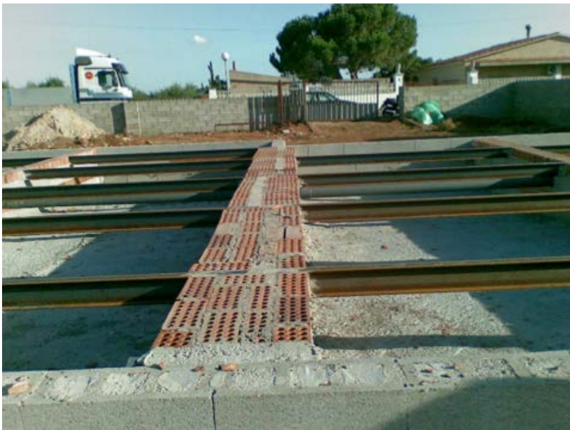
Figure 4. Suspended floor structure.
