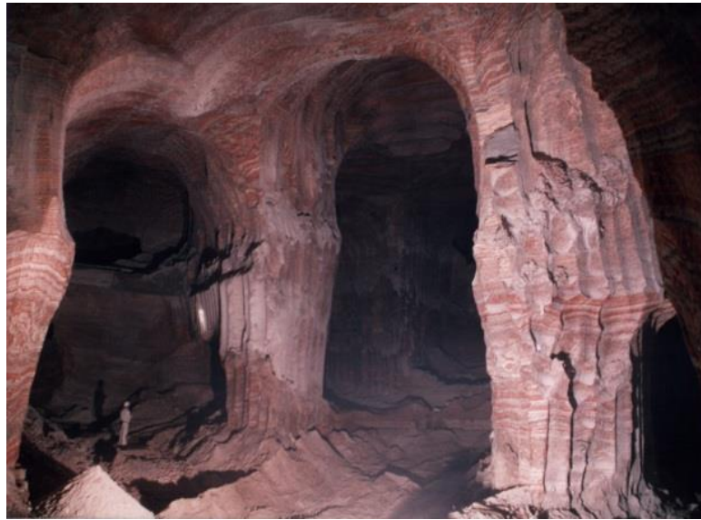
Figure 3. Image of some pillars in a potash mine (Source: ICL Iberia).
