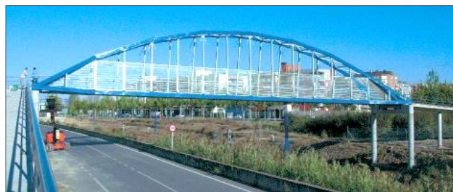
Figure 2.9: General view of the all-FRP footbridge from Lleida, Spain [19].
