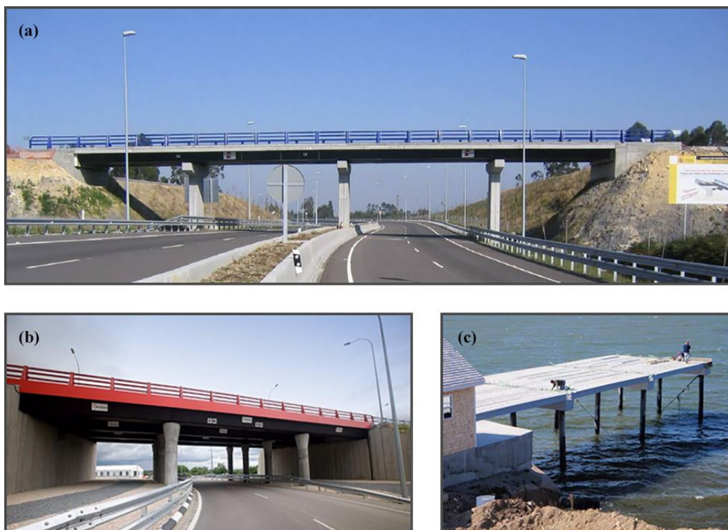
Figure 2.11: Examples of infrastructure projects incorporating hybrid FRP-concrete beams: (a) the Cantábrico highway overpass bridge; (b) the M-111 highway overpass bridge (both images courtesy of ACCIONA Infraestructuras); (c) the marine pier of the Downeast Institute for Applied Marine Research and Education (courtesy of Downeast Institute).
