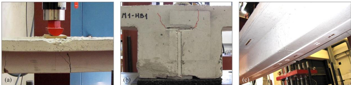
Figure 3.30: Failure characteristics of hybrid beams model M1 in test setup I: (a) concrete crushing and flexural cracks; (b) inward slip and flange delaminations; (c) bottom flange separation.
