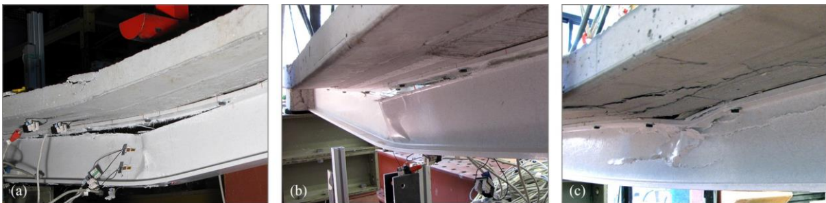
Figure 3.31: Failure characteristics of hybrid beams model M2 in test setup I: (a) profile web-flange shear delamination preceded by concrete slab crushing; (b) post-failure local buckling of the web; (c) transverse crushing of the profile's web.
