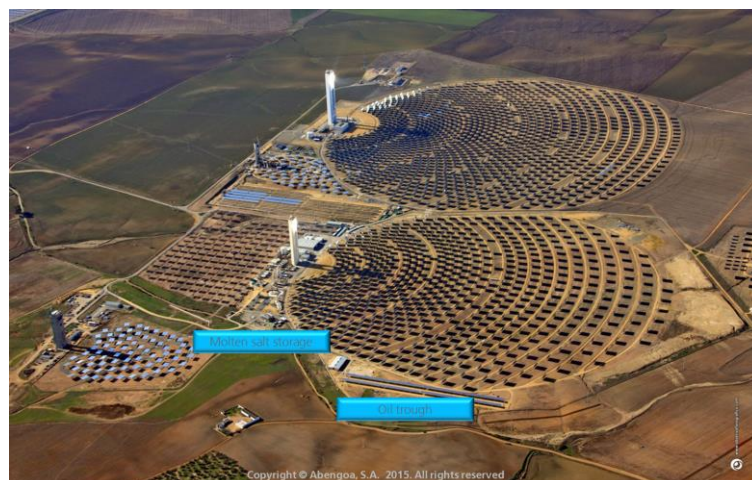
Figure 13 Solúcar Solar Platform of Abengoa (Sevilla, Spain)
