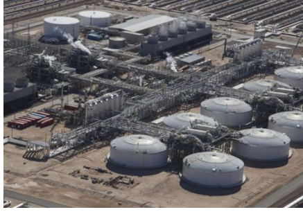
Figure 5. Molten salt storage of Solana Plant (Abengoa, Arizona, 250 MW)
