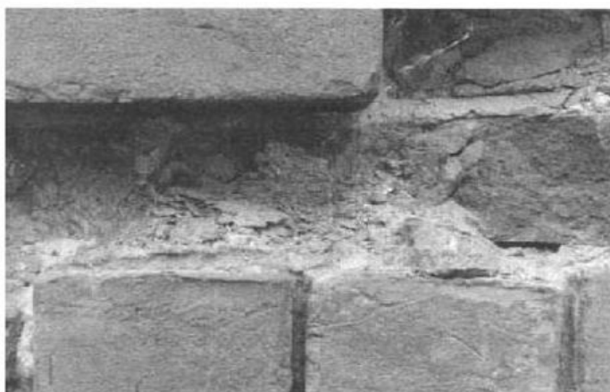
Figure 9 Free-thaw processes have caused these construction bricks in Ouray, Colorado, to break apart (from Schiffer 1987: 183, Figure 7.6).
