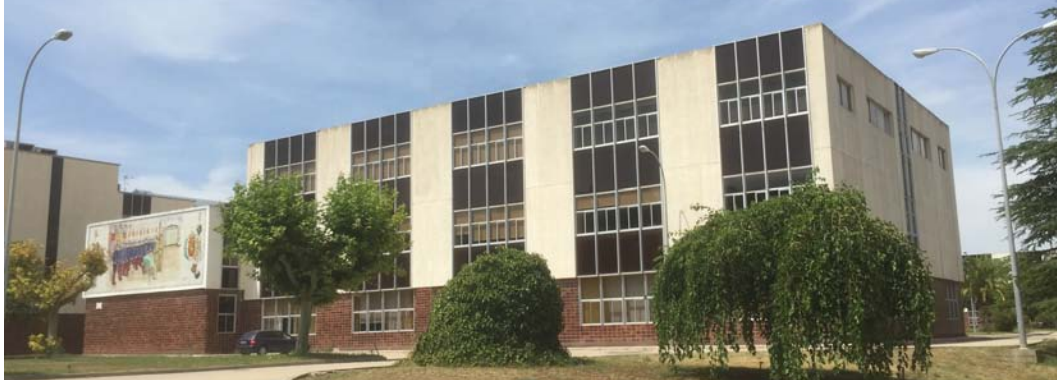
Figure 2.8. General view of the building under study
