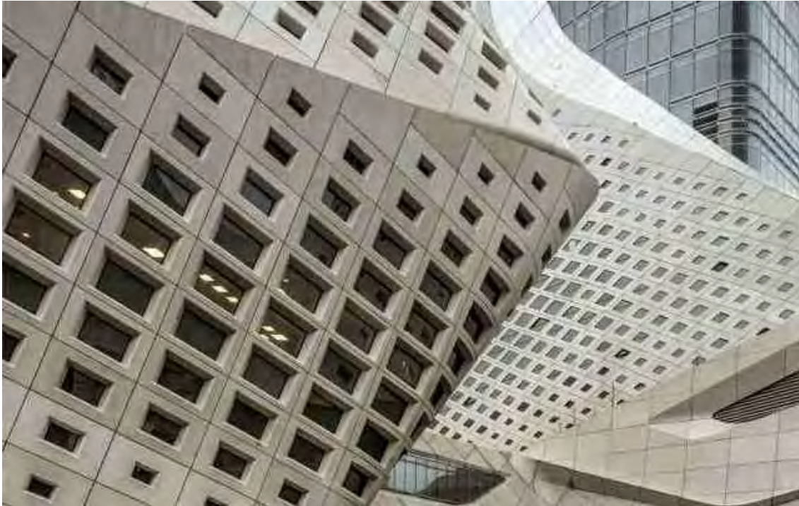
199 Zaha Hadid Architects, Nanjing Youth Olympic Centre, Nanjing, 2011
