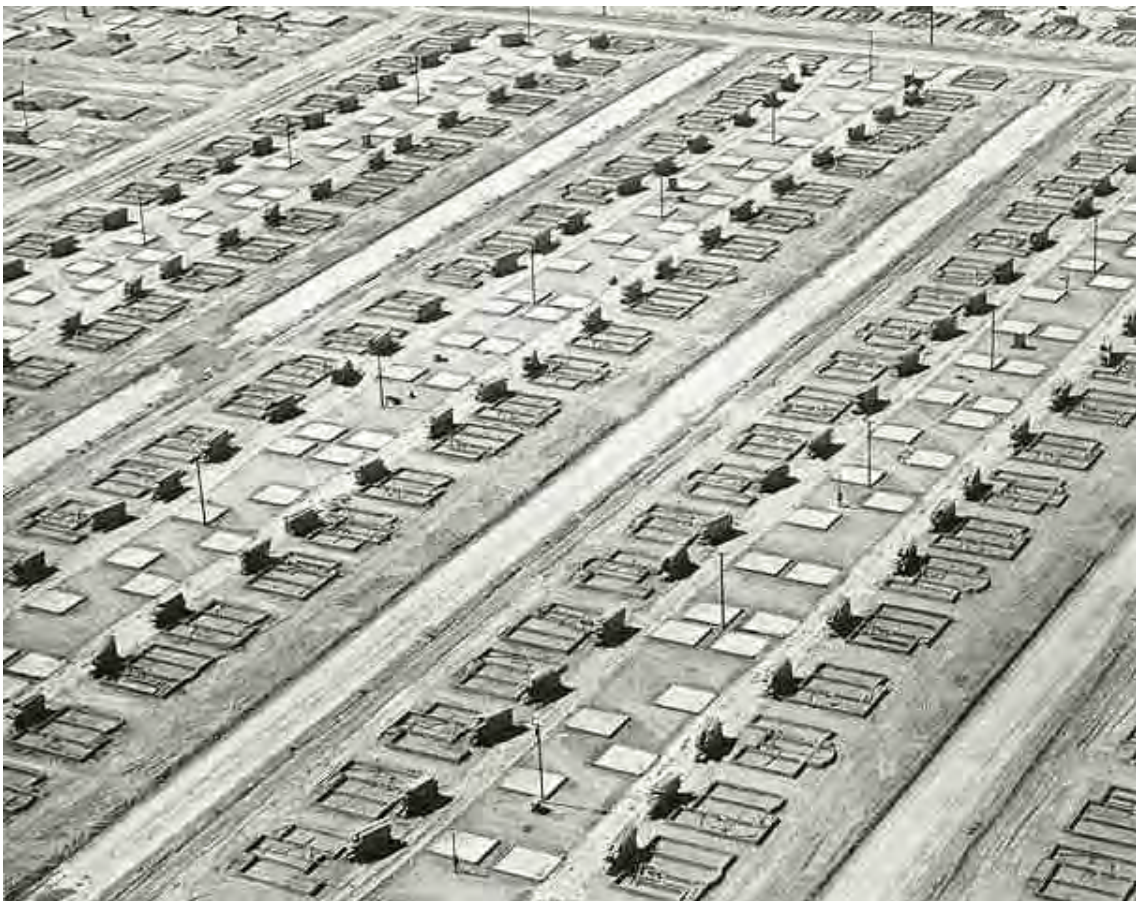
93 William Garnett. "Foundations and slabs, Lakewood, California", 1950
