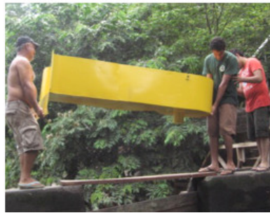
[6.8] Installation of an axial “Simplex” in León, Nicaragua 2012 (author’s photos)
