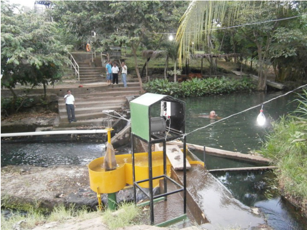
[6.9] Installation of axial “Simplex” Turbine in León Nicaragua 2012, (author’s photos)
