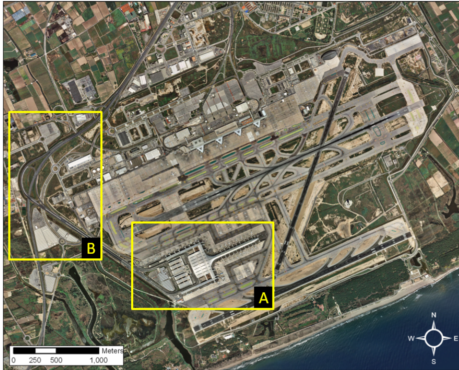
Figure 3.2: General overview of Barcelona-El Prat airport. The areas of interest selected are the terminal T1 (A) and the access road (B).
