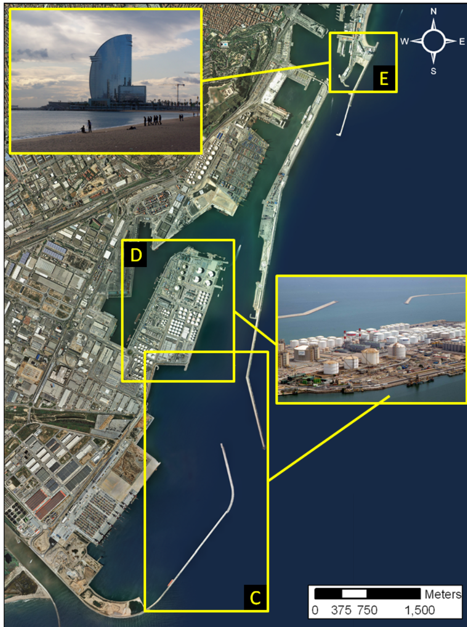
Figure 3.3: General overview of El Port de Barcelona. The areas of interest selected are the breakwaters (C), the Energy Bay (D) and W Barcelona hotel (E).
