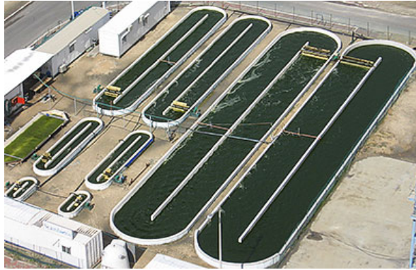
Figure 1.1 Microalgae open reactors (raceway systems). An aerial view of a pilot plant (Seambiotic Ltd., Tel Aviv) growing Nannochloropsis (an algae are rich in oil) using flue gas CO 2 from a coal-fired Power Plant near Ashkelon, Israel. Small ponds used to inoculate the largest (Seibert, 2009).
