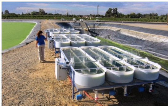
Figure 7.2 Real view of triplicate South, Middle and North high rate algal ponds of Delhi facilities.
