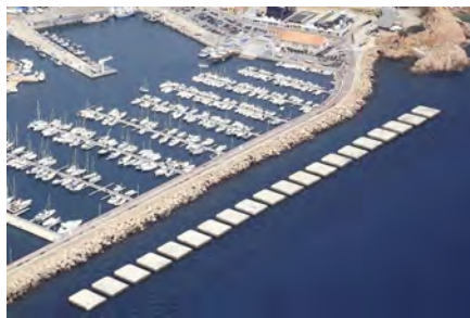
(a) Breakwater structure
