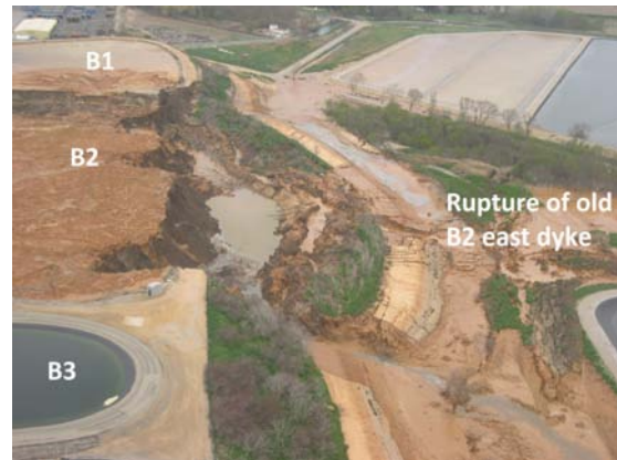
Figure 2.9: Aerial view of the B1, B2 and B3 basins showing the rupture of the B2 eastern dyke, March 2004 (Source: AREVA).
