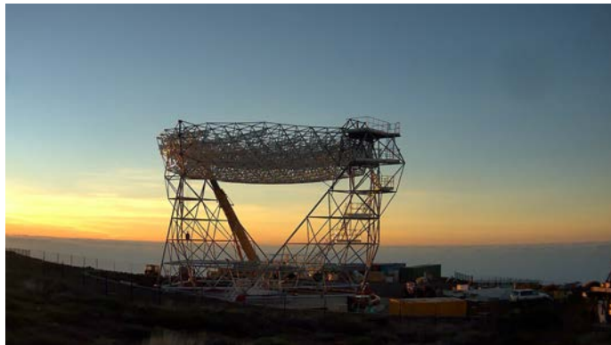
Figure 3.23: Picture taken on 4 th of December from LP by Javier Herrera . It was taken during the LST1 operation of lifted the mirror dish on top of the understructure.
