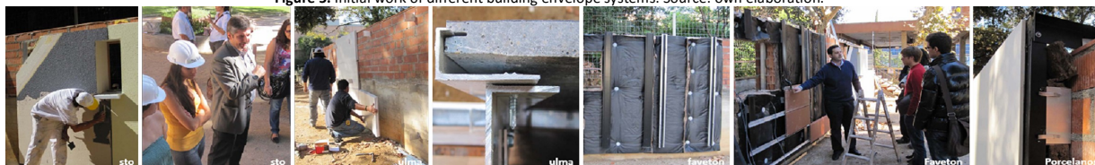
Figure 5. Initial work of different building envelope systems. Source: own elaboration.
