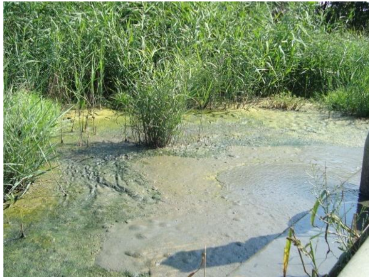
Figure 10.4 Vegetation growth problems in Alpens (on the top) and in Santa Eulalia (on the bottom), Spain.
