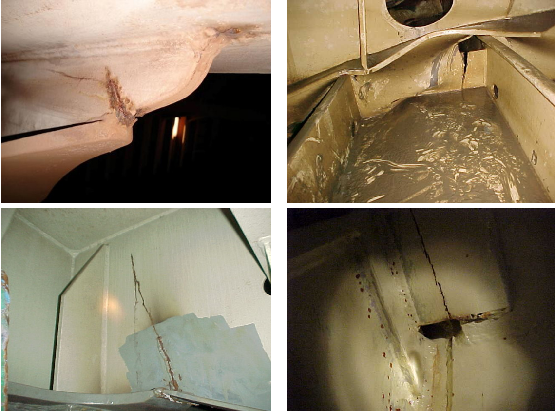
Figure 4.17: Examples of cracks on vessels structures.
